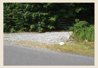
fall off the tires before the vehicle leaves the site. Periodic maintenance maybe required to keep the tracking pad clean and in working condition.
