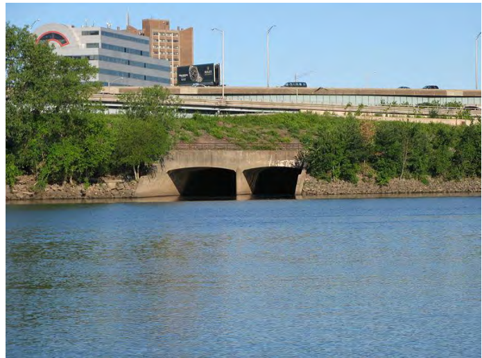
The confluence of the Park River conduit with the Connecticut River in Hartford.
