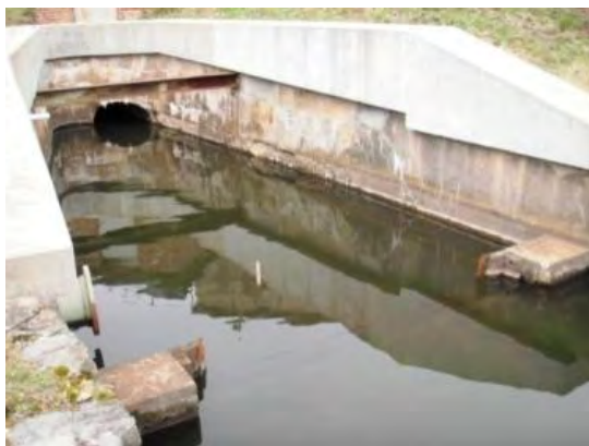
Figure 6-11. North Stamford Dam low flow outlet
