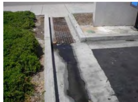
Figure 6-34. Wash water from a commercial car wash discharging down a storm drain is an example of an illicit discharge. Source: EPA
