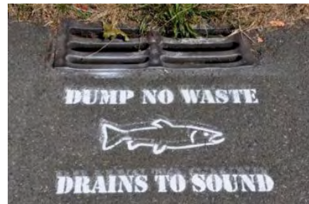
Figure 6-29. Example of storm drain stencil. Source: Unknown
