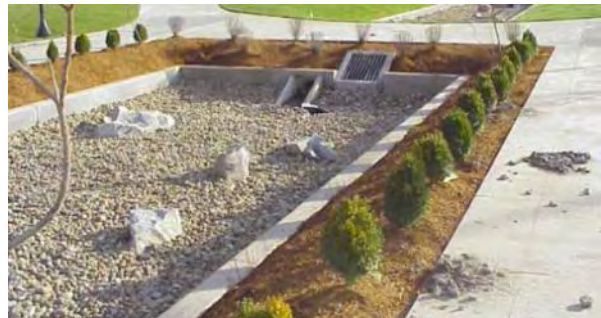
Figure 6-9. Sand Filter in an urban park. Source: Unknown.
