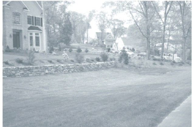
Figure 6.4.20 – Vegetative filter strip. Source: Connecticut, 2004.
