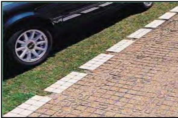
Figure 6.4.17 – Permeable pavement. Source: Connecticut, 2004.
