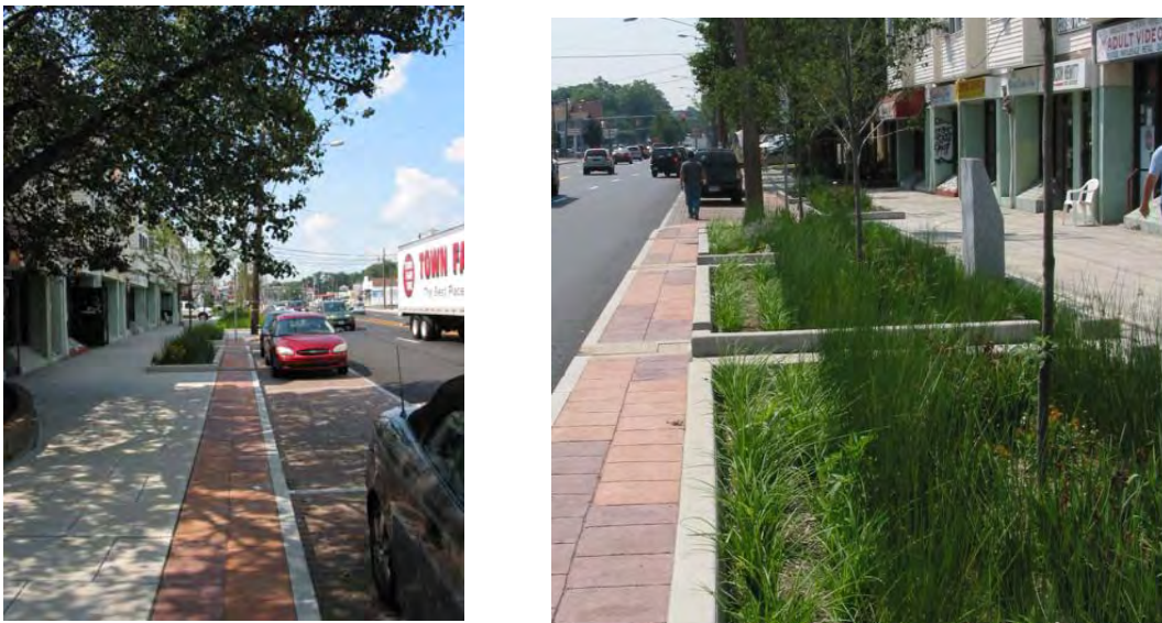
Figure 6.3.12 – Permeable pavement (left photograph) and rain garden/bioretenion (right photograph) retrofits along North Main Street in Bridgeport, CT.
