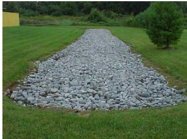
Figure 6.4.30 – Infiltration trench.
