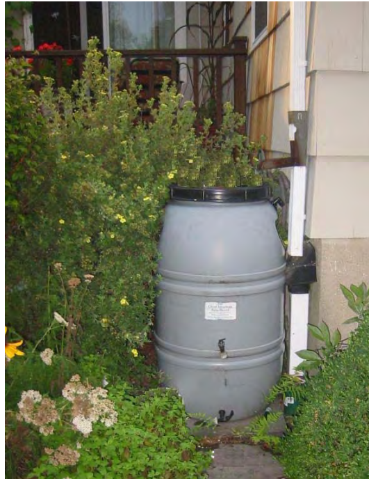
Figure 6.4.26 – Example of a rain barrel. Source: Connecticut Department of Environmental Protection.
