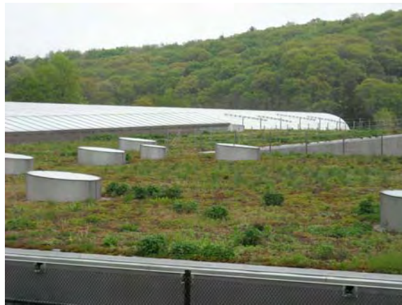
Figure 6.3.16 – Retrofit and redevelopment techniques in Connecticut. Source: Connecticut Department of Environmental Protection.
