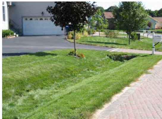
Figures 6.4.22 – Vegetated drainage way. Photograph courtesy of the University of Connecticut NEMO program, Kara Bonsack
