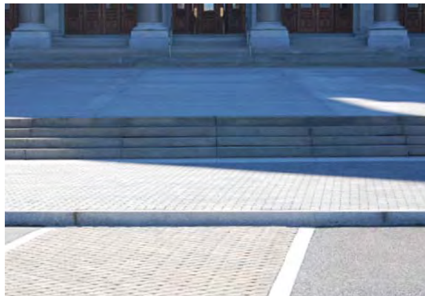
Figure 6.3.15 – Permeable pavement at Hartford Green Capitols Project. Source: Camp Dresser & McKee.
