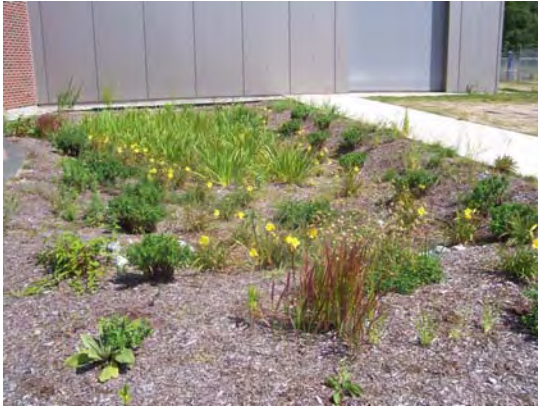
Bioretention area at University of Connecticut Storrs Campus.
