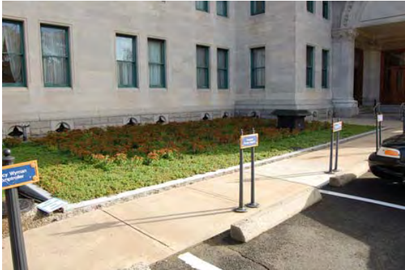
Figure 6.3.13 – Green roof at Hartford Green Capitols Project. Source: Camp Dresser & McKee.
