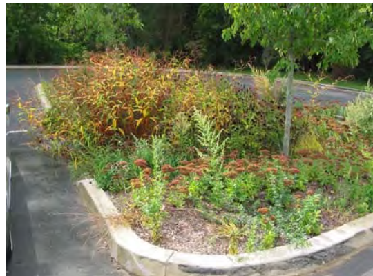
Figure 6.4.15 – Bioretention in use as a parking lot island in Branford, CT. Source: Connecticut Department of Environmental Protection.
