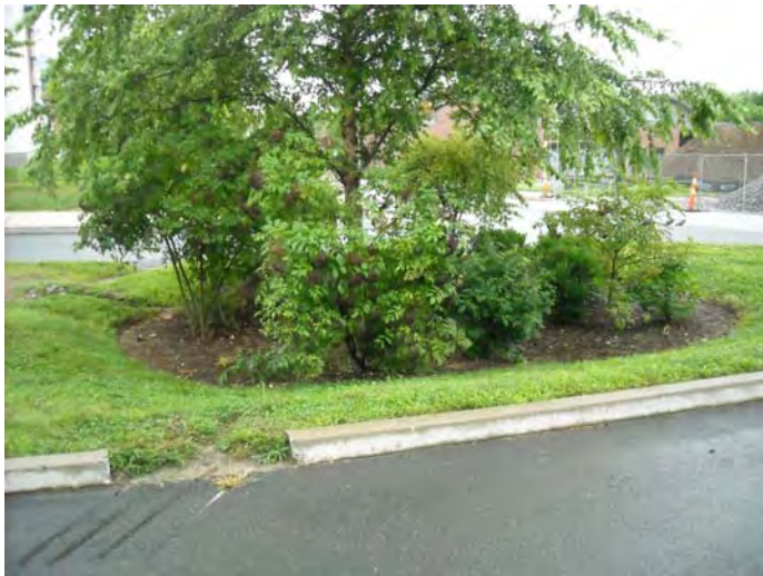
Figure 6.4.28 – Bioretention at University of Connecticut Storrs Campus –Mansfield, CT. Source: Connecticut Department of Environmental Protection.
