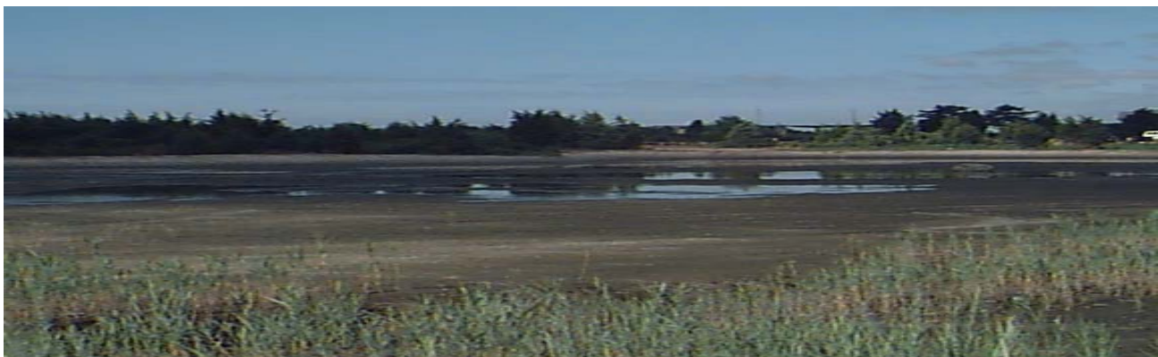
Western segment immediately following the removal of sandy dredged sediment at low tide. Small pond in the background and a section of excavated creek in the lower right (area 3).
