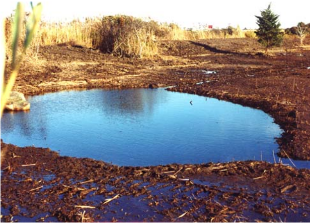
Meig Point wetland (area 2). Shows the wetland immediately following the removal of the Phragmites dominated fill area and a small excavated pond.
