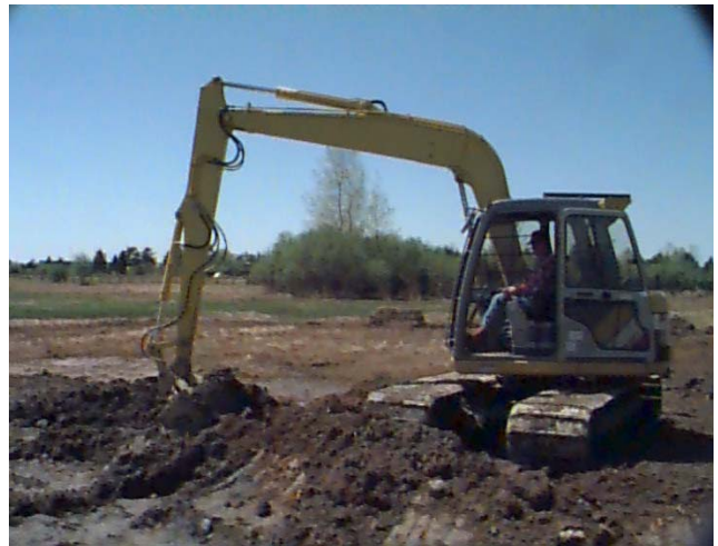
Cleared ditch (area 1)
