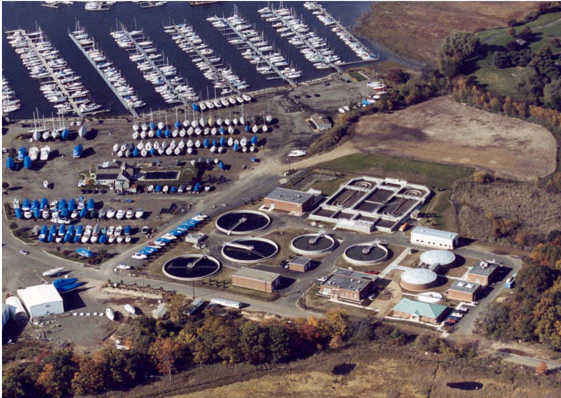
Branford, Connecticut Wastewater Treatment Facility*
