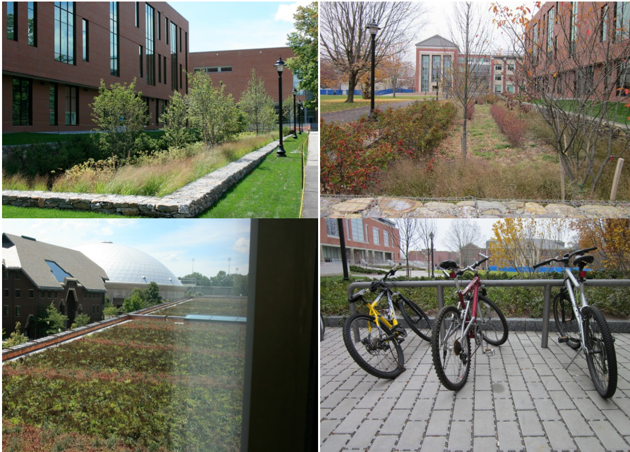
Figure 3: Low impact development practices installed in 2011 at UCONN's new West Classroom Building: top left – bioretention swale in summer, top right – bioretention swale in fall, bottom left – green roof, bottom right – porous pavers. (CLEAR, 2012)
