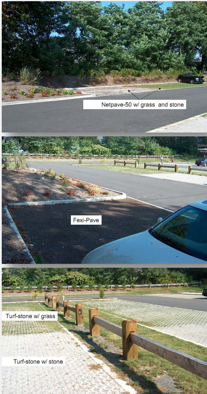
Figure 3: Examples of the different types of pervious parking lots installed at the Hole-in-the Wall Outdoor Classroom. (NFWF, 2009b)
