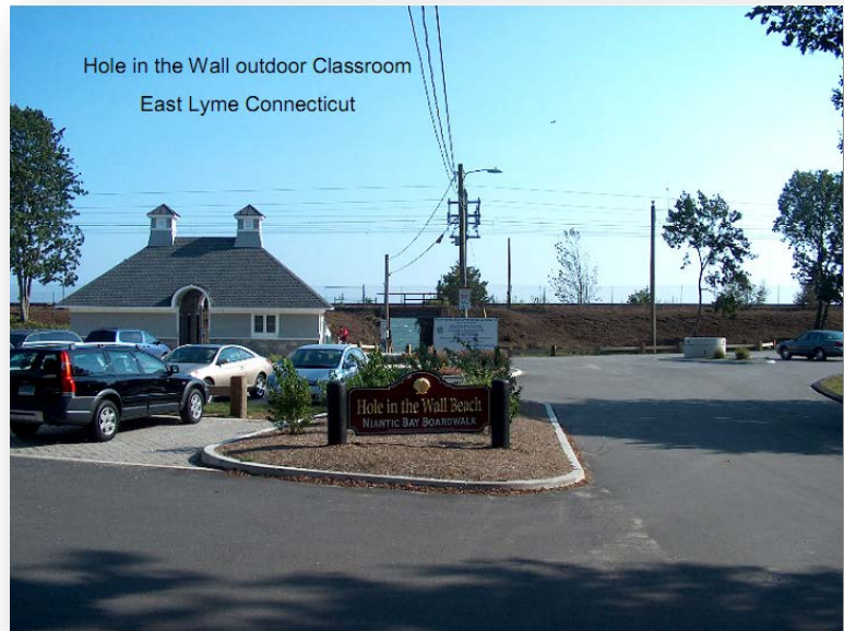
Figure 2: The Hole-in-the Wall Outdoor Classroom. (Town of Lyme)
