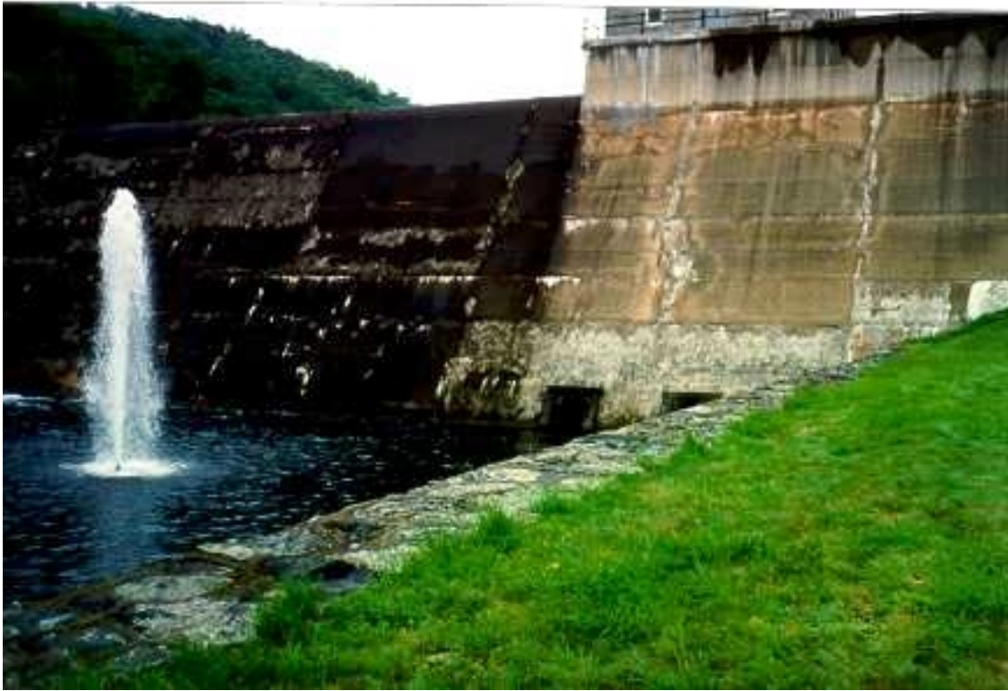
Shepaug Dam on the Shepaug River, Warren / Litchfield border, CT. Impoundments and dam structures such as this can be used to make releases to maintain streamflow during low flow periods.
