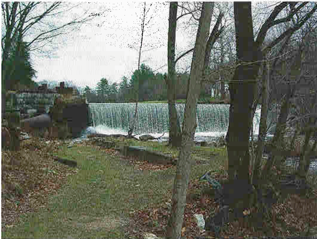
Lower Pond Dam at the John Beckley Furnace (Canaan No. 2) site.
