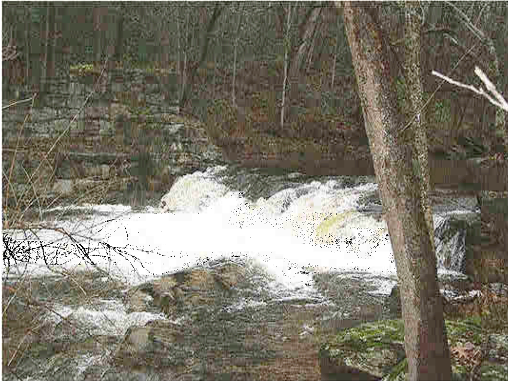
The unnamed dam at the former Samuel F. Adam Furnace (Canaan No.1) site.
