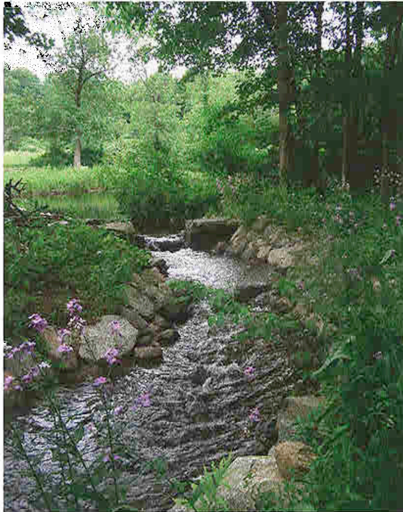
Cannondale Dam Bypass Channel, Norwalk River, Wilton
