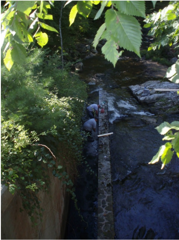
Figure 7. Cutting out the bottom of the existing Fishway.
