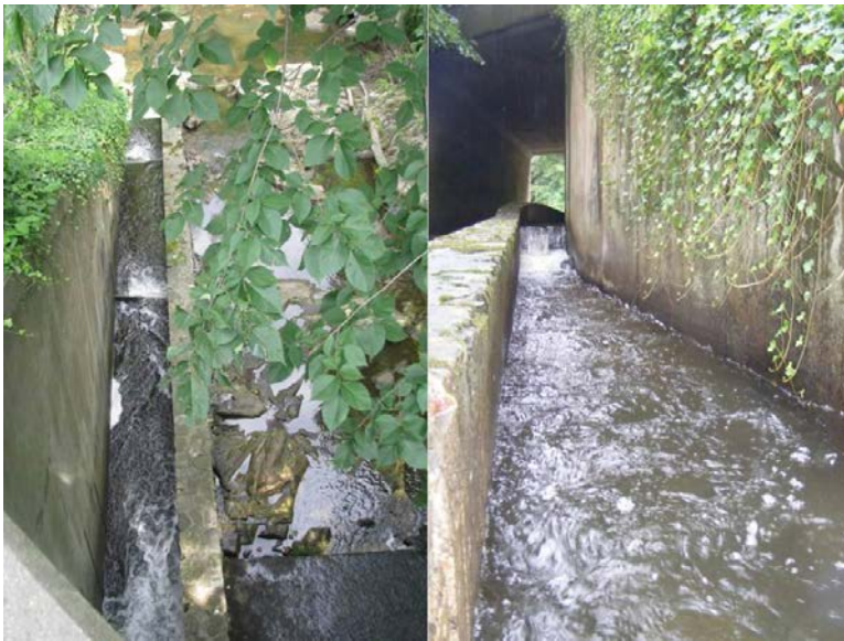
Figure 4. Two pre-construction views of the interior of the fishway. There was no internal flow control, consequently the flows inside the fishway were too fast for fish to pass through.
