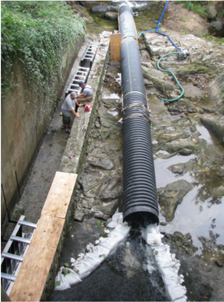
Figure 9. Positioning the three Steeppass units
