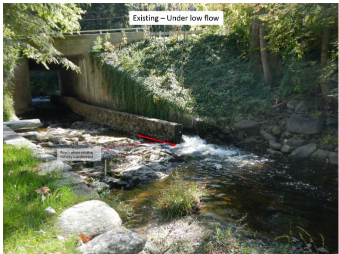
Figure 1. Pre-construction conditions of the fishway
