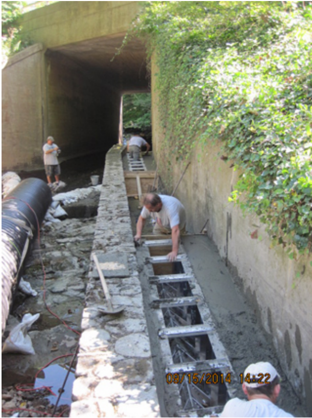
Figure 10. Installing the Steeppass units (September 15, 2014)
