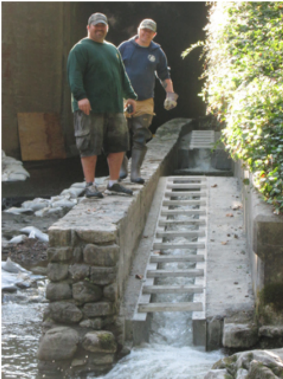
Figure 11. Completed fishway
