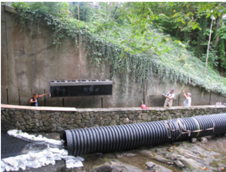
Figure 8. Lowering down an Alaskan Steeppass unit
