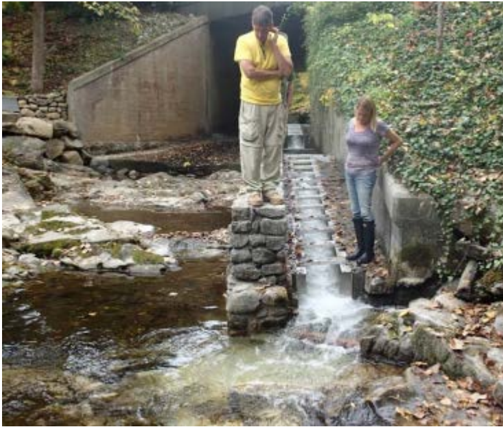
Figure 12. Tim Wildman (IFD) and Laura Wildman (design engineer with Princeton Hydro) observe the lower portion of the refurbished fishway.
