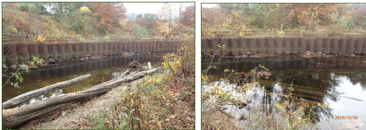
Downstream (left) and cross-stream (right) views of the reconfigured log jam.
