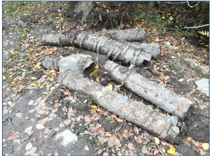
Banded wooden pipe removed (and replaced) from the well field at Burlington Hatchery.
