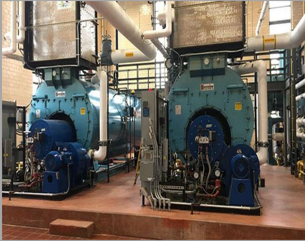
Figure 12: New central power plant boilers installed
