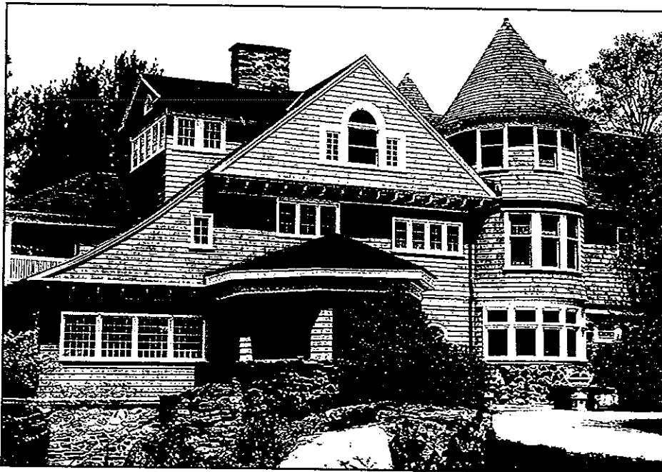
12. Erik Rossiter House (The Rocks), Washington Green Historic District, Washington. Shingle style, 1888-1889. View north.
