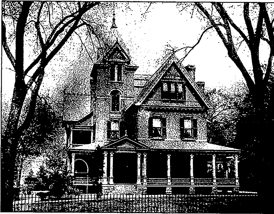
9. Bronson Tuttle House, Naugatuck. Historic photograph, Queen Anne style, 1879-1881. View west.
