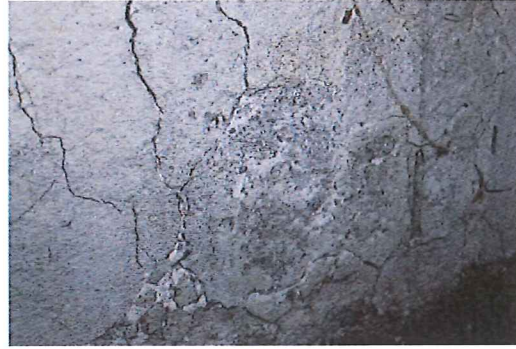
(c) map cracking
