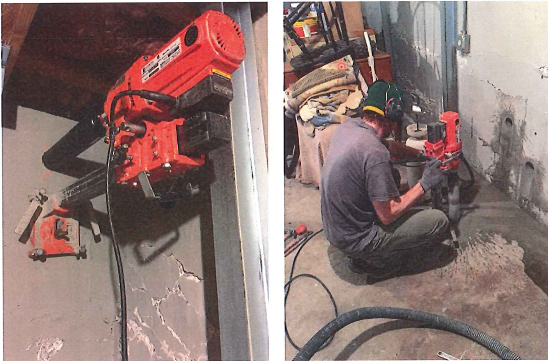
Fig. 4.1 Coring process carried out by a third party contractor
