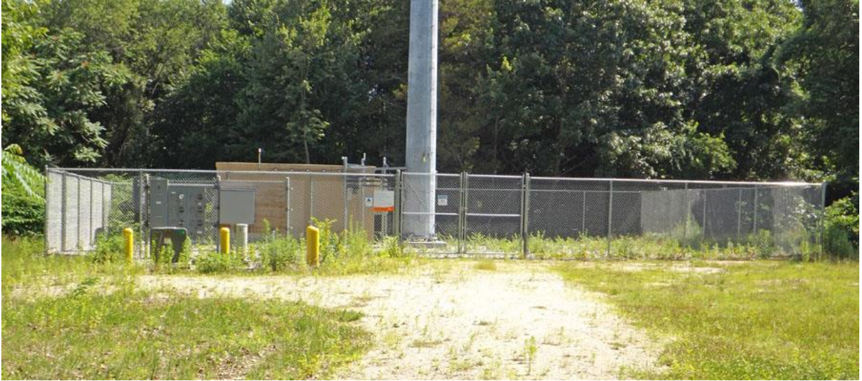
View of base compound
