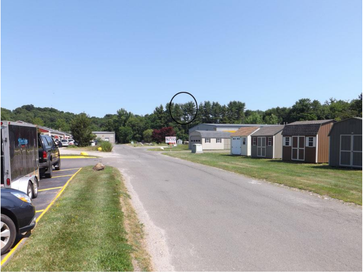
View of tower near Route 1
