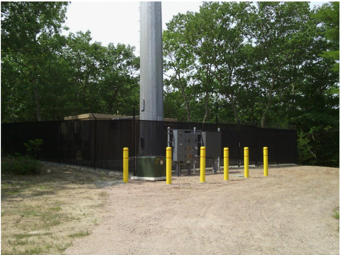
Compound view – NE corner.
