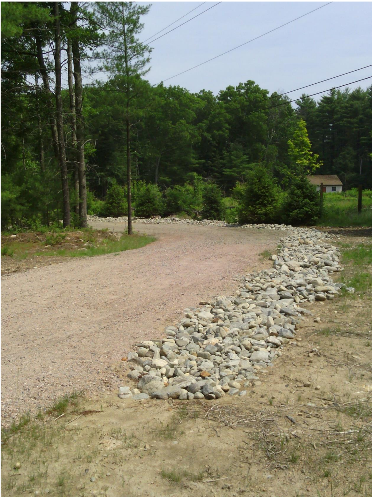
Access road drainage ditch. Note new plantings along curve to screen site from lessor's residence.
