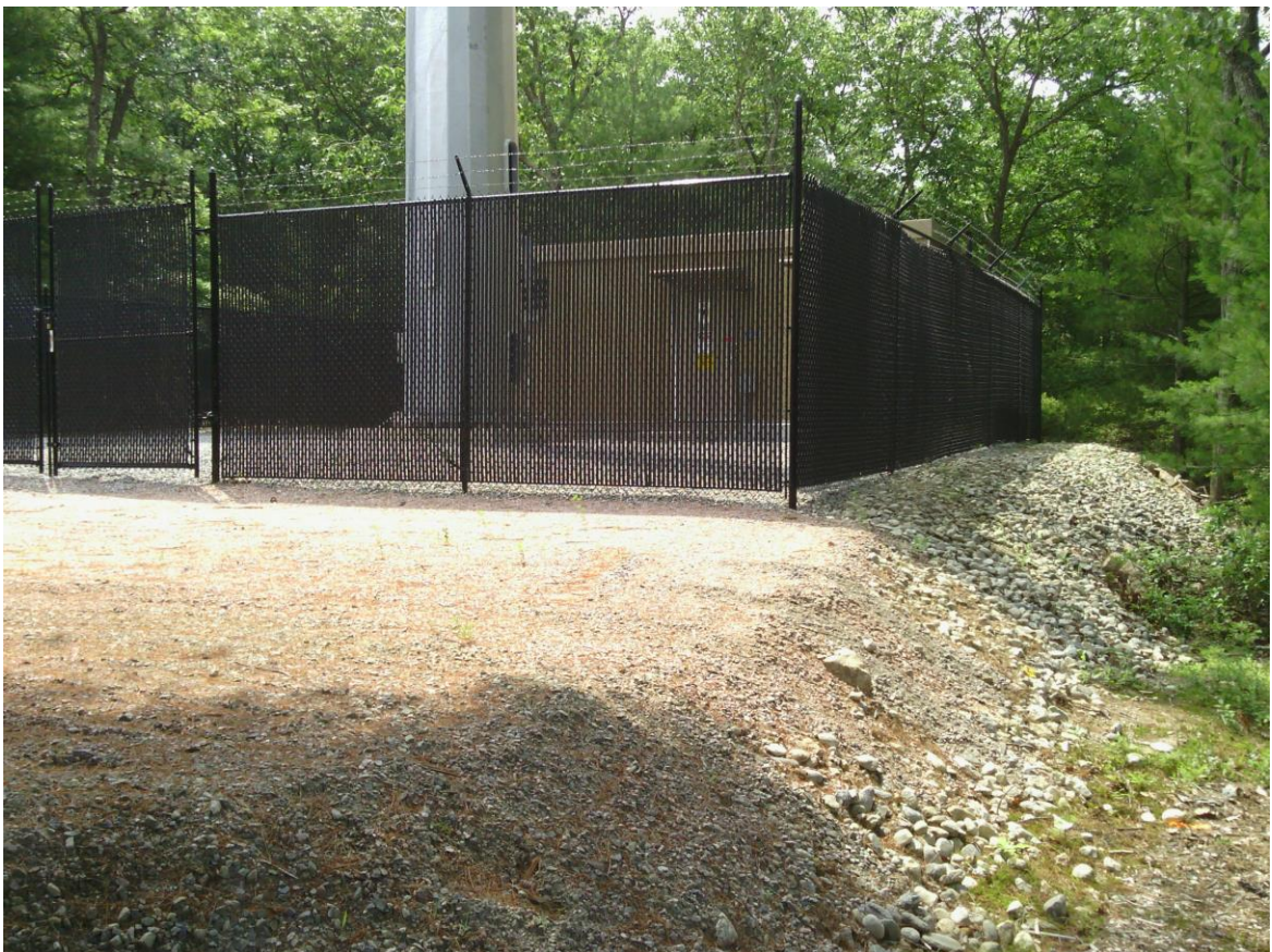
Compound view – NW corner.
