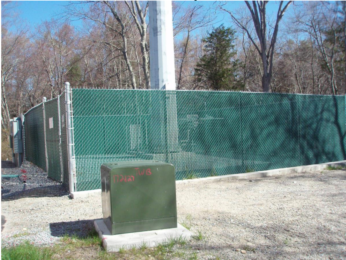
View of base compound
