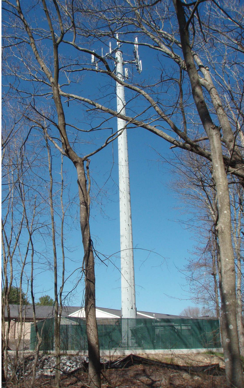
View of tower
