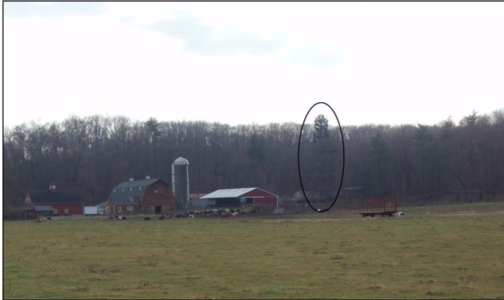
View of tower from Town Farm Road, looking southwest
