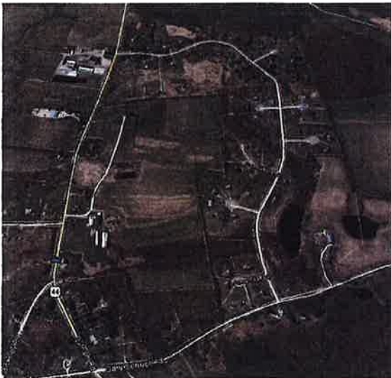
Longmeadow Estates (67 lots) is the largest single family development in Town. Amara Farm is located at the top left of the aerial photo.
