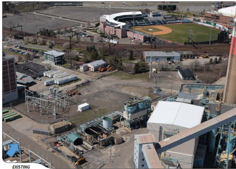
Figure 4-6: Representative View of Proposed Substation Site and Immediate Vicinity
