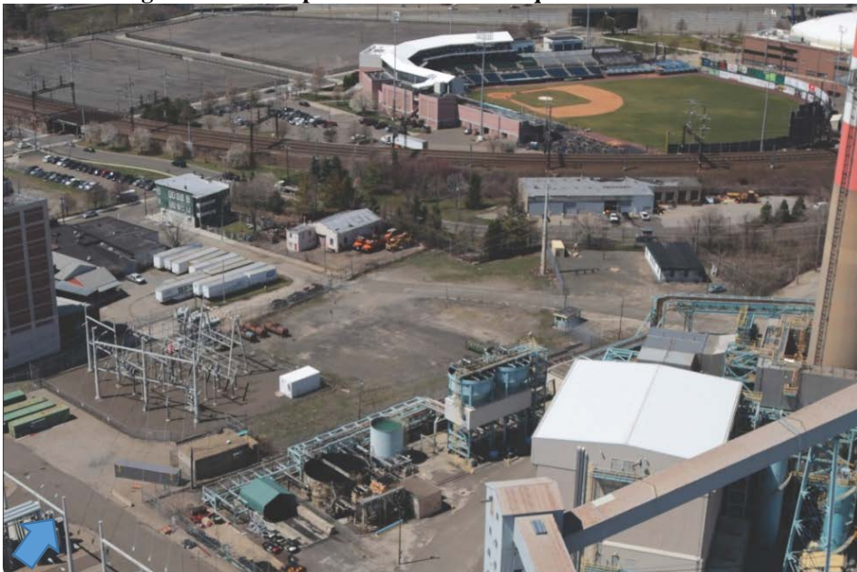
Figure ES-2: Proposed Site for New Pequonnock Substation
