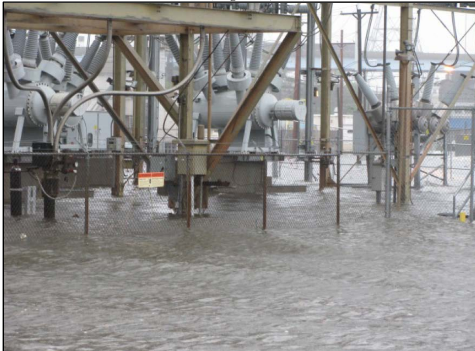
Figure 1-4: Photograph of Coastal Flooding at Existing Pequonnock Substation during Tropical Storm Irene (August 28, 2011)
