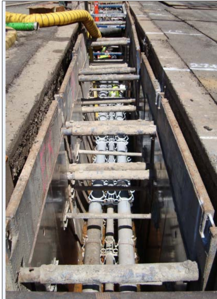
Figure 3-2: Typical XLPE Duct Bank Construction in Road
