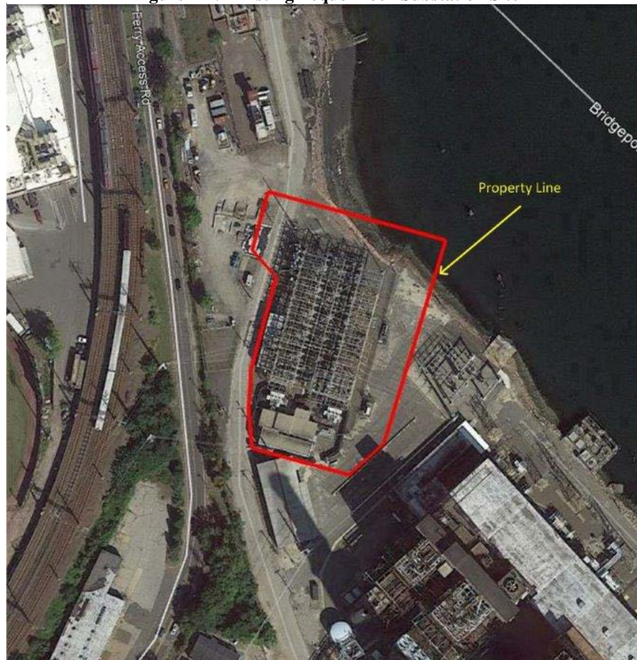
Figure 1-2: Existing Pequonnock Substation Site
