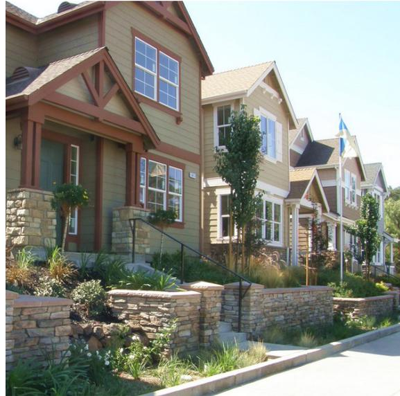
Flow-through planters are hard-edged stormwater management facilities with an impermeable base, and are appropriate where infiltration of stormwater is unsafe or not possible—typically urban environments. They treat water by allowing runoff to soak through a soil matrix and filter into an underdrain system.
