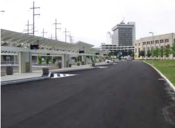
Inter-modal Center (front view) | Source: Stantec
