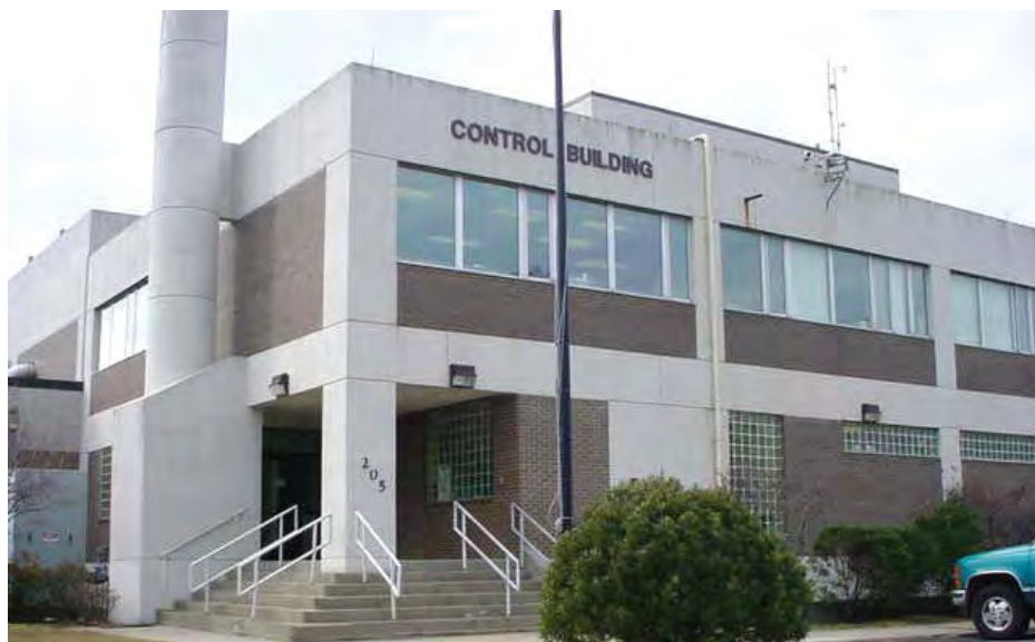
WPCA Treatment Plant | Source: City of Bridgeport
