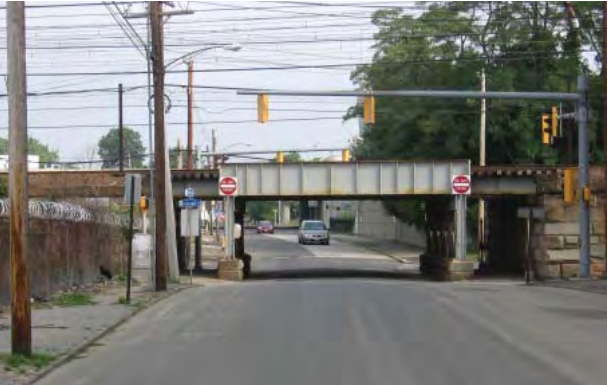
New Haven Rail Line | Source: Stantec
