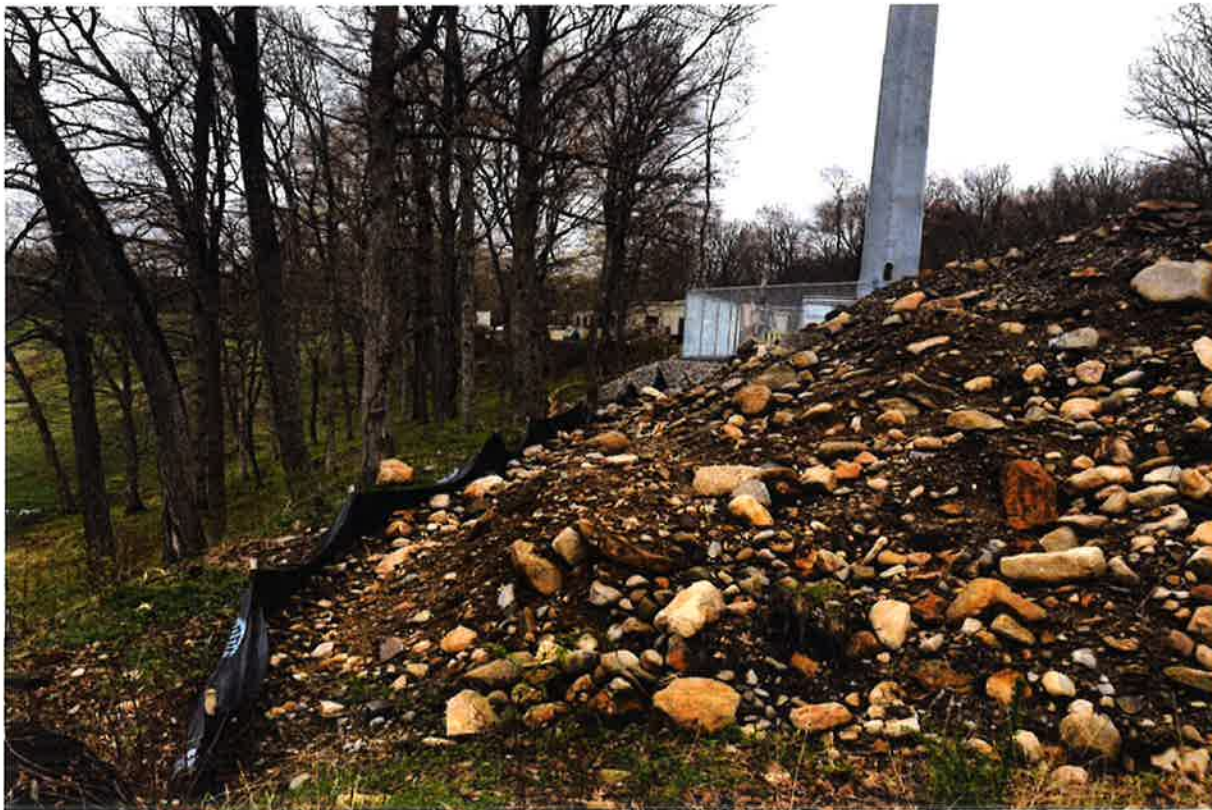
Photo 6: View of temporary excavation stockpile.
