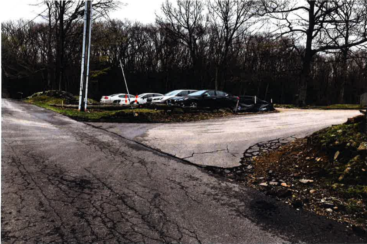
Photo 1: View of construction entrance off Folly Lane.
