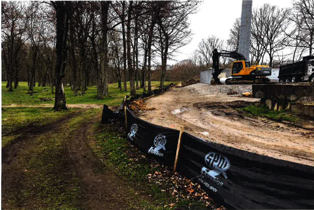
Photo 5: View of E&S perimeter controls adjacent to bulk storage bins.
