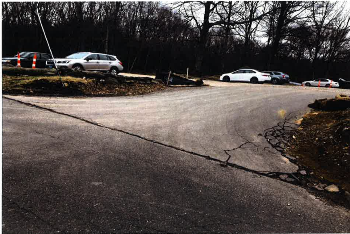
Photo 1: View of construction entrance off Folly Lane.
