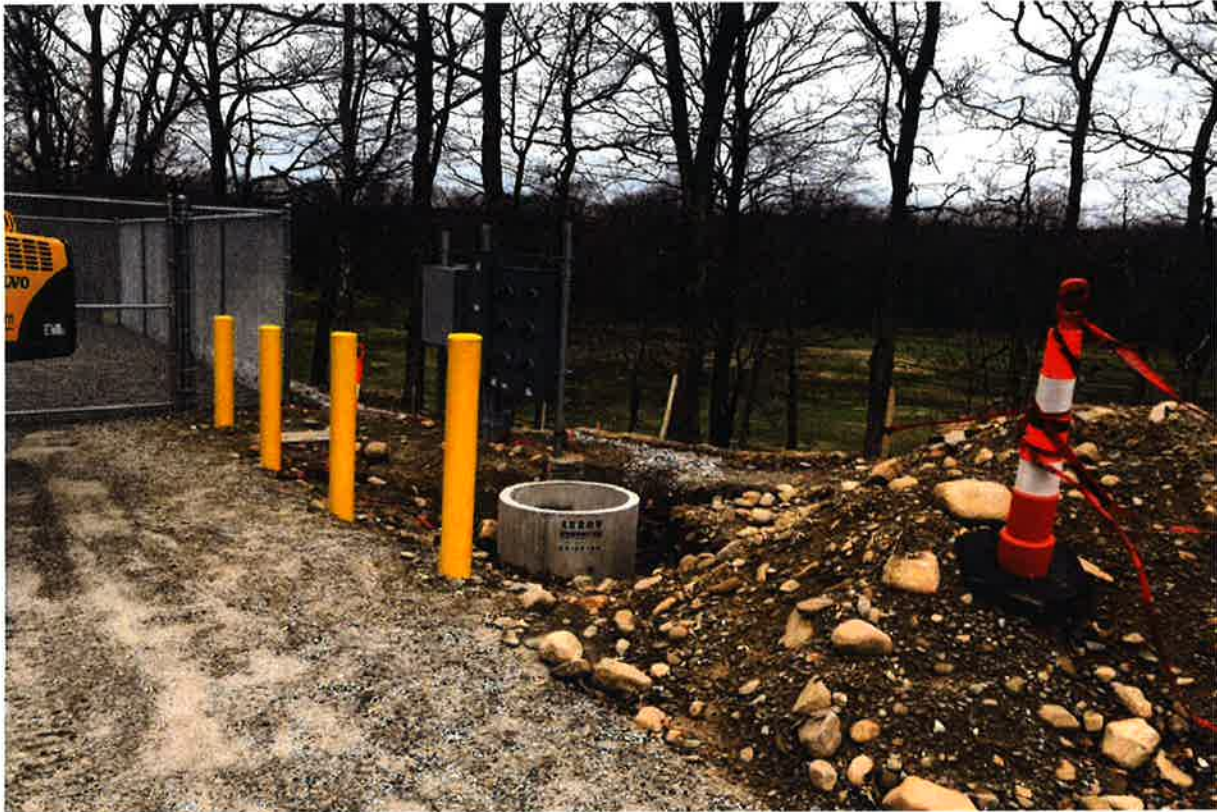
Photo 3: View of ongoing electrical work adjacent to compound area.
