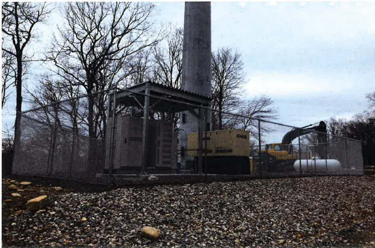
Photo 2: View of compound area.
