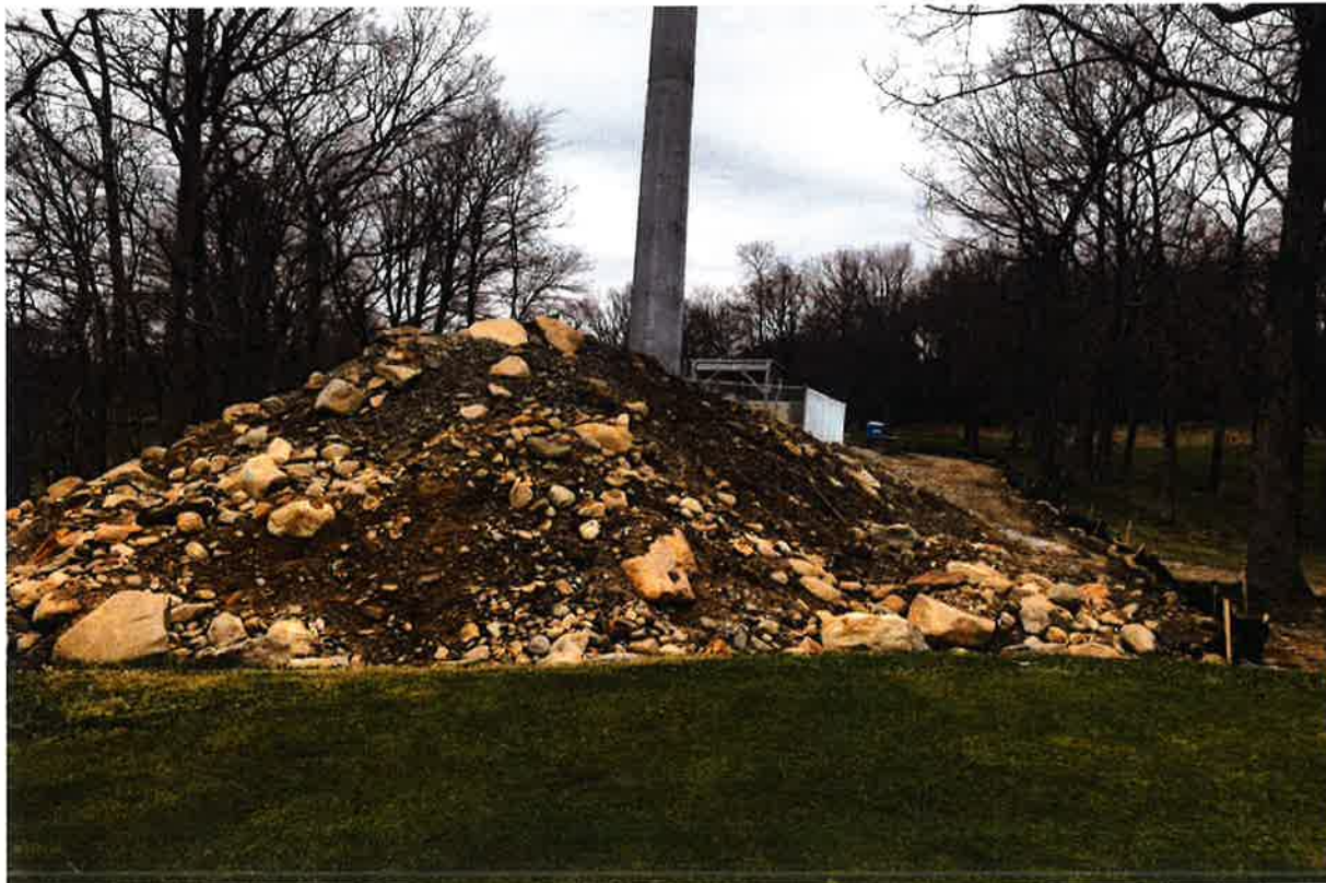
Photo 6: View of temporary excavation stockpile.
