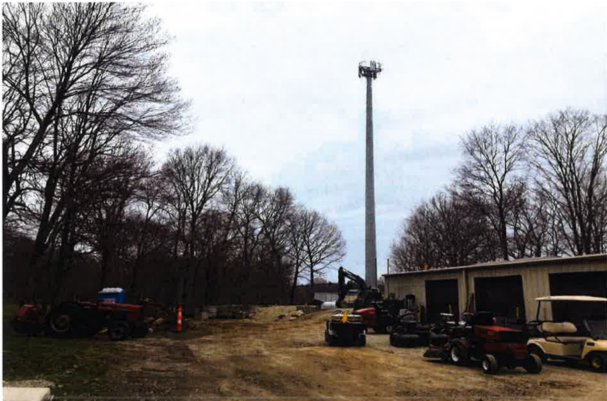
Photo 4: View of access road to compound area and tower.
