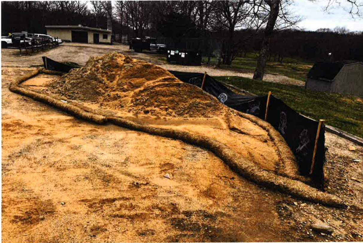
Photo 5: View of material storage pile.
