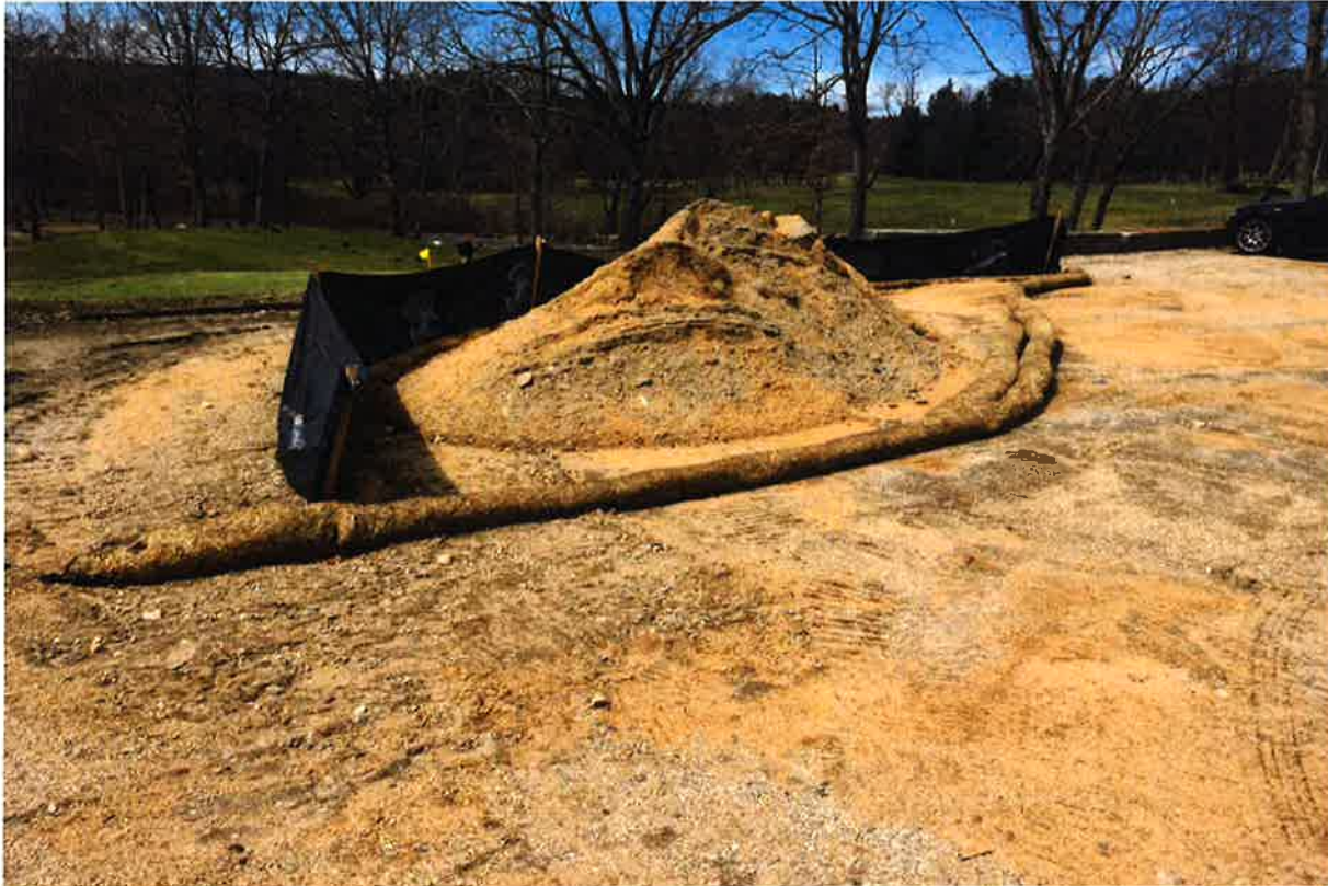
Photo 5: View of material storage pile.
