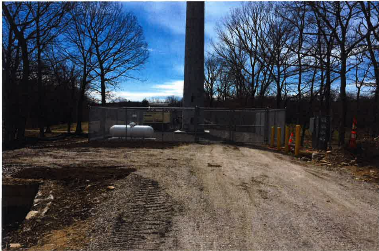
Photo 4: View of compound area.
