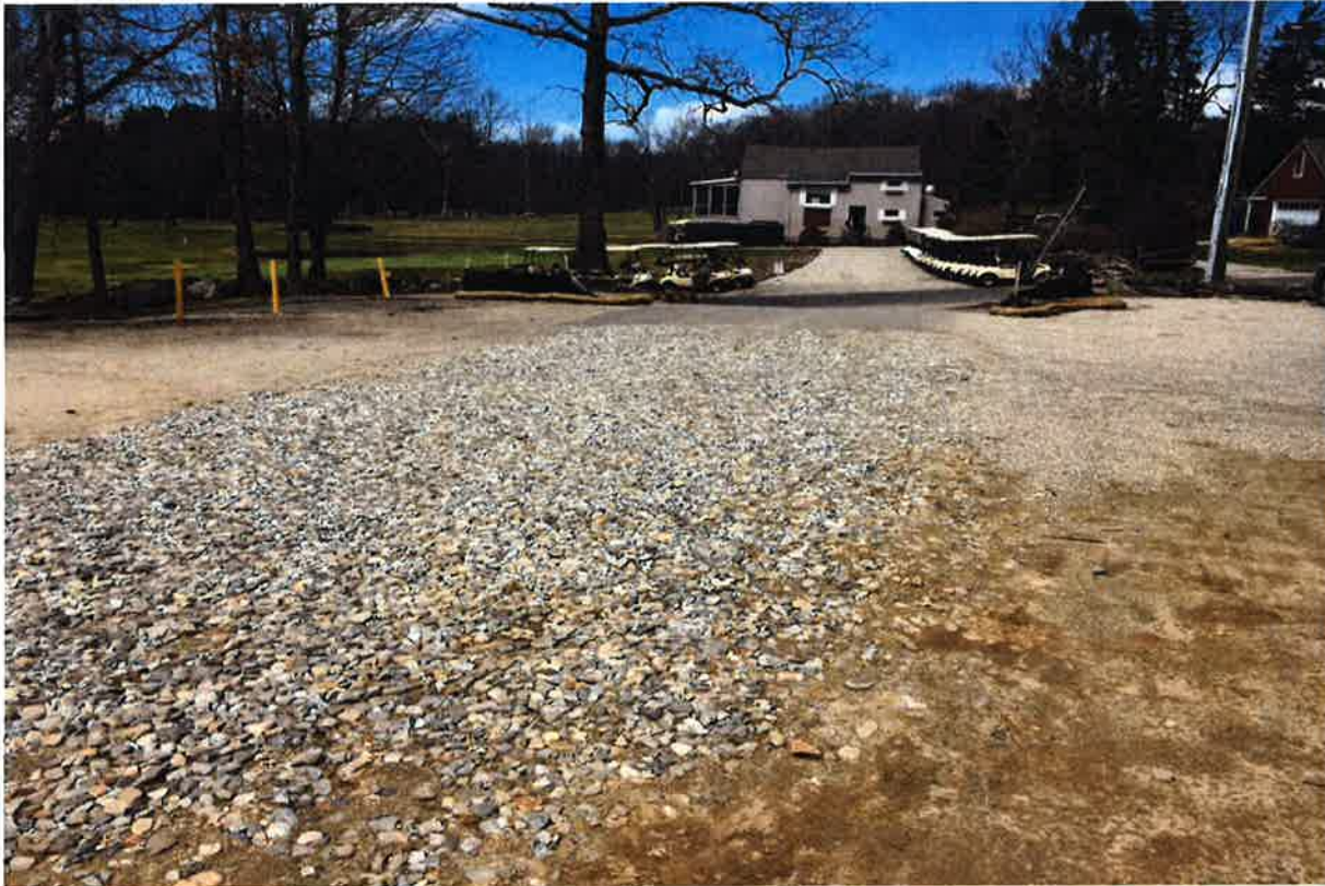
Photo 1: View of construction entrance off Folly Lane.
