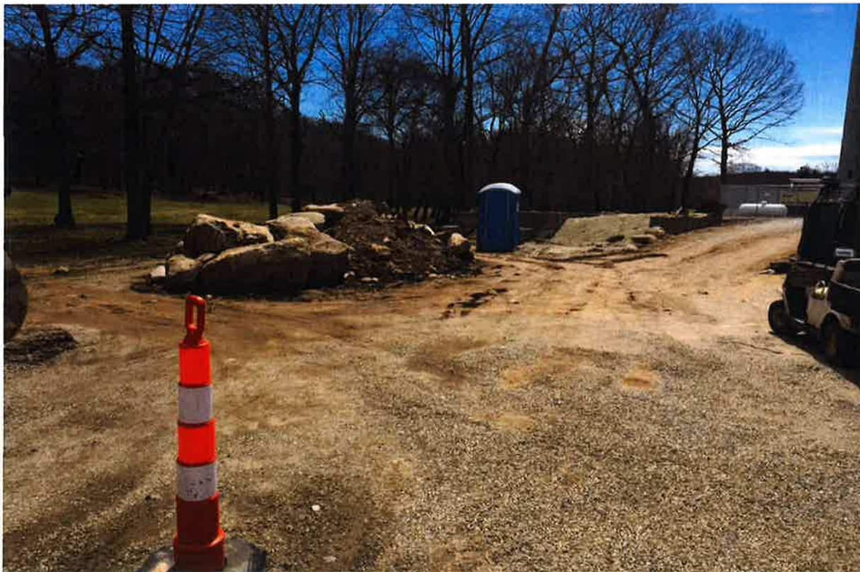
Photo 6: View of temporary stockpile adjacent to bulk storage bins.
