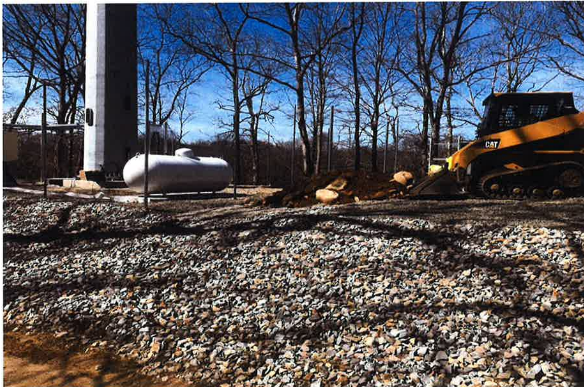
Photo 4: View of compound area under construction.
