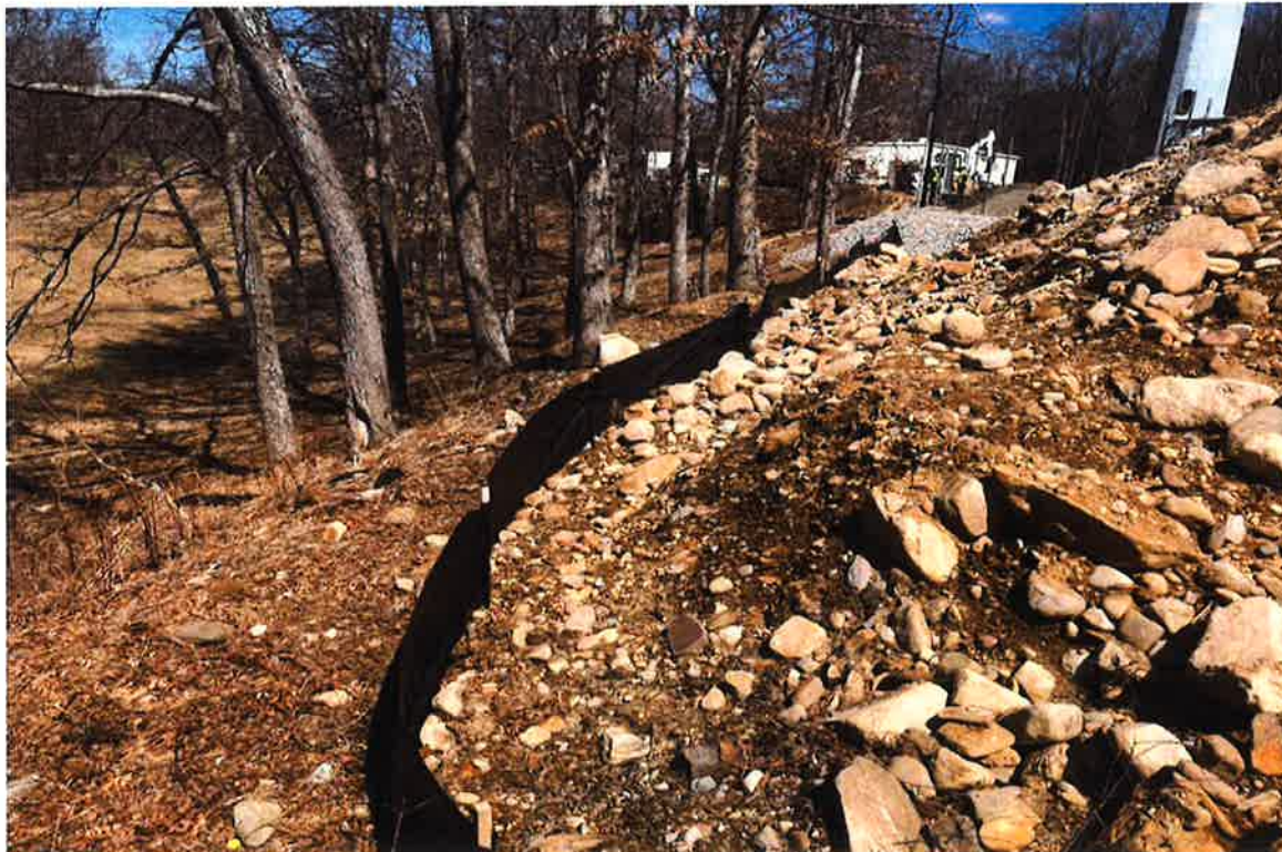
Photo 6: View of excavation material pile.
