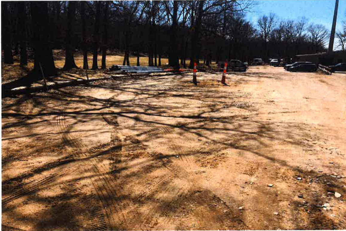
Photo 5: View of trenching area filled in.
