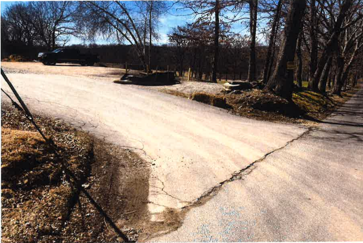
Photo 1: View of construction entrance off Folly Lane.
