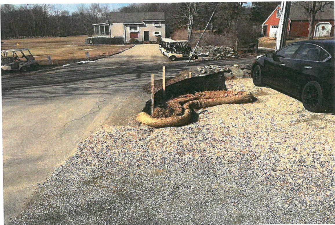
Photo 2: View of repaired/reinforced E&S controls at construction entrance.
