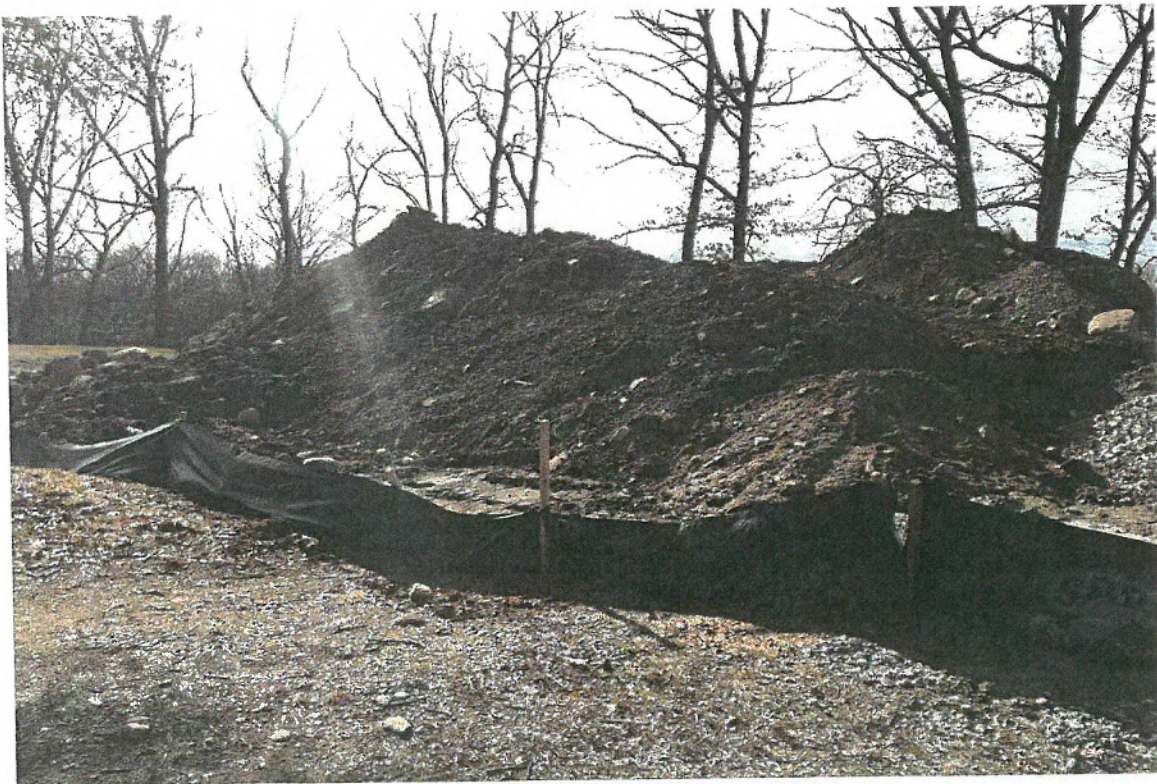
Photo 6: View of excavation material pile.
