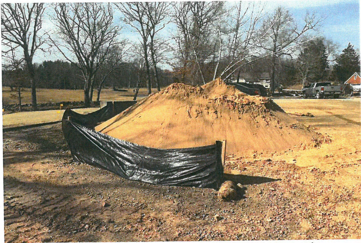
Photo 5: View of material storage pile with maintained perimeter controls.
