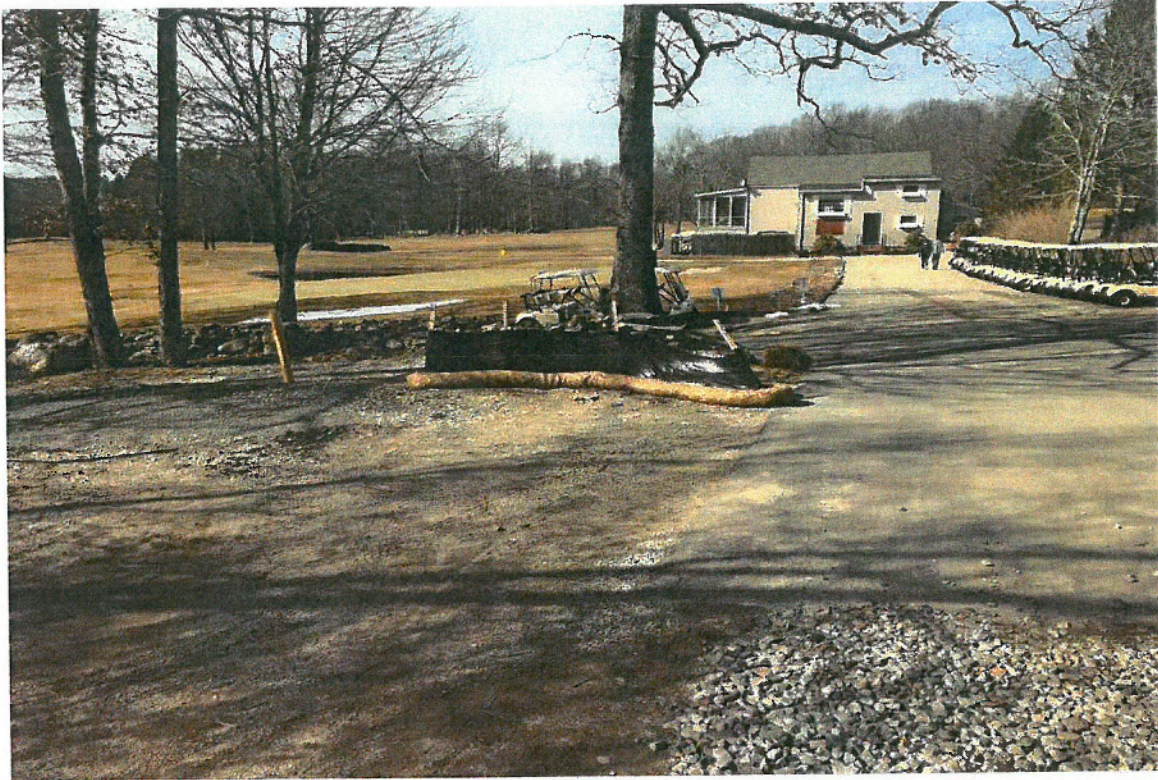
Photo 1: View of construction entrance off Folly Lane.
