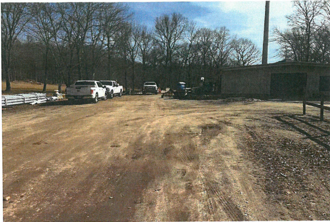
Photo 3: View of access road.
