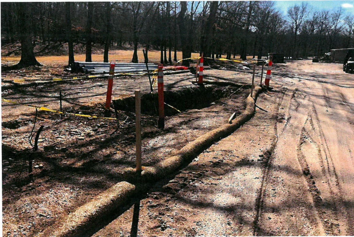
Photo 7: View of straw wattle along trenching.
