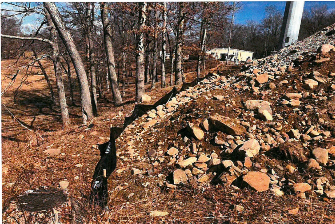
Photo 4: View of excavation material pile.
