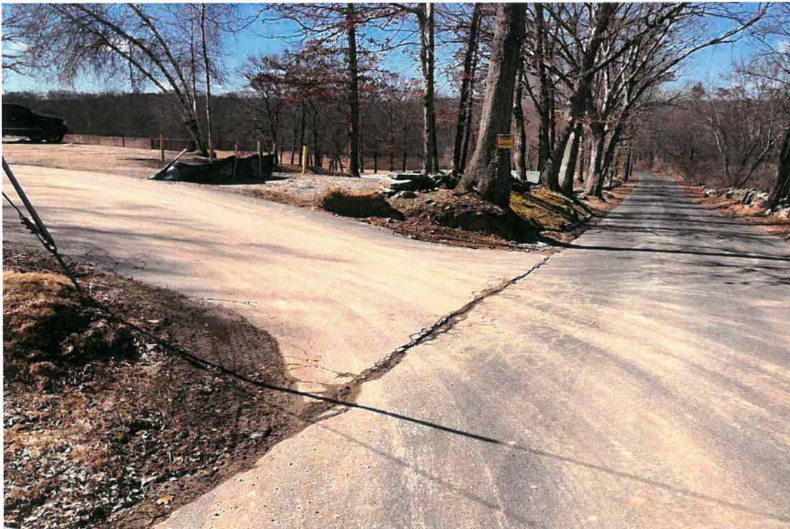
Photo 2: View of E&S controls at site entrance.
