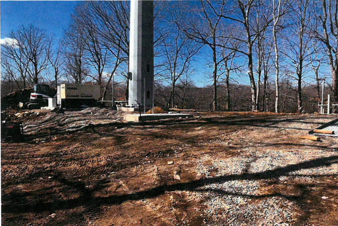
Photo 3: View of ongoing tower work.
