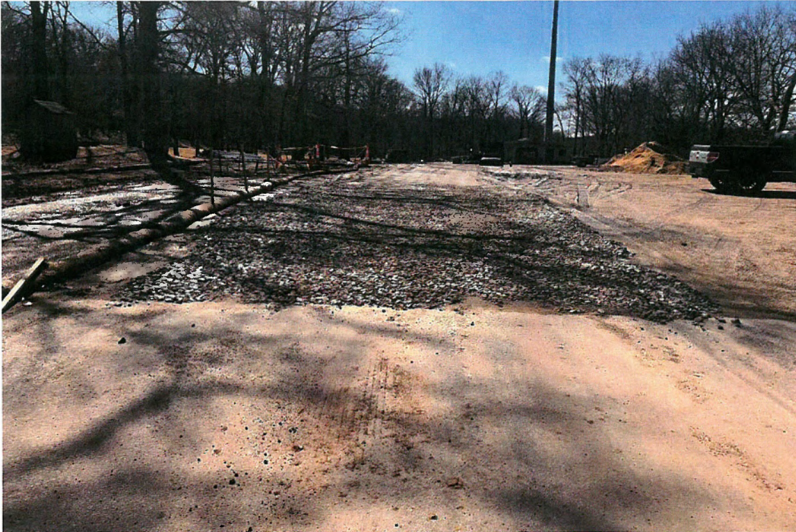
Photo 1: View of tracking pad at construction entrance off Folly Lane.
