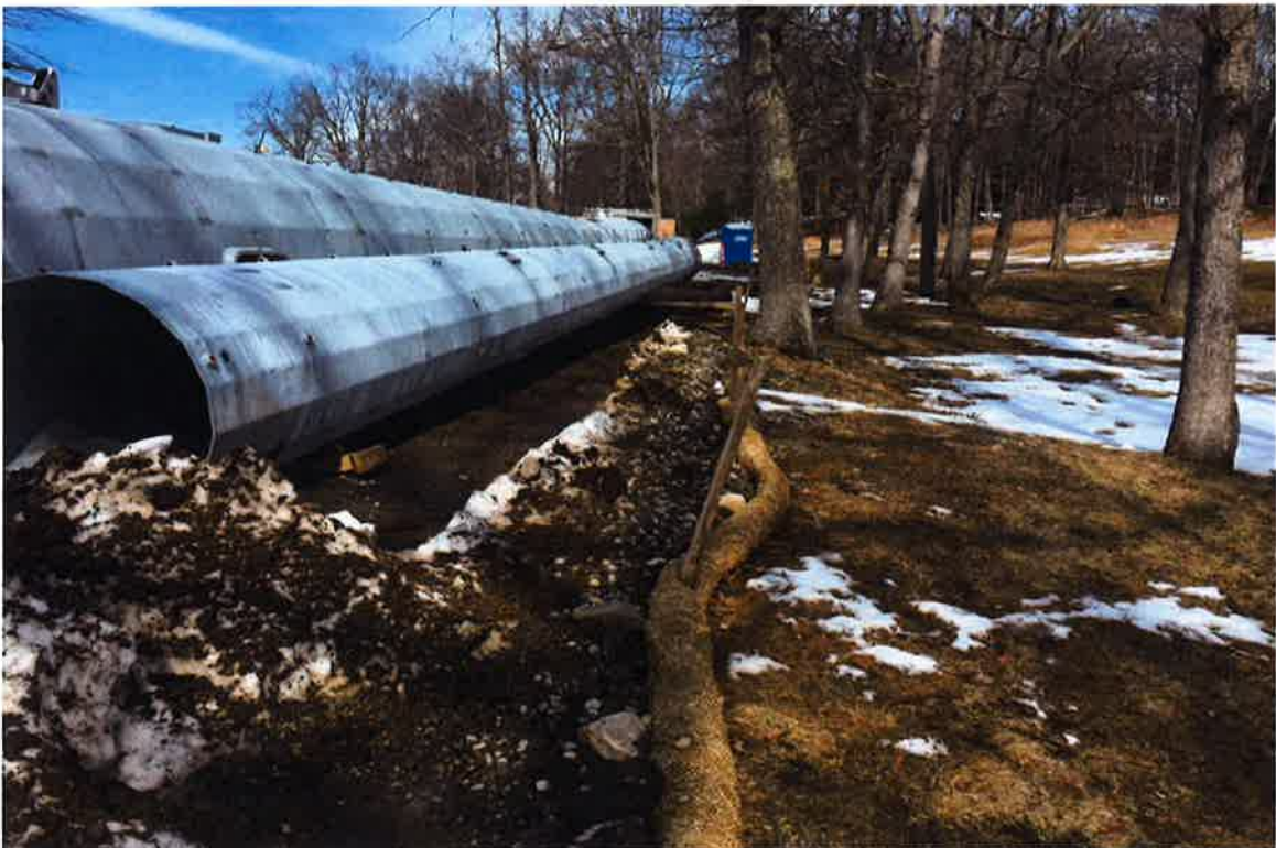
Photo 4: View of staged tower sections.
