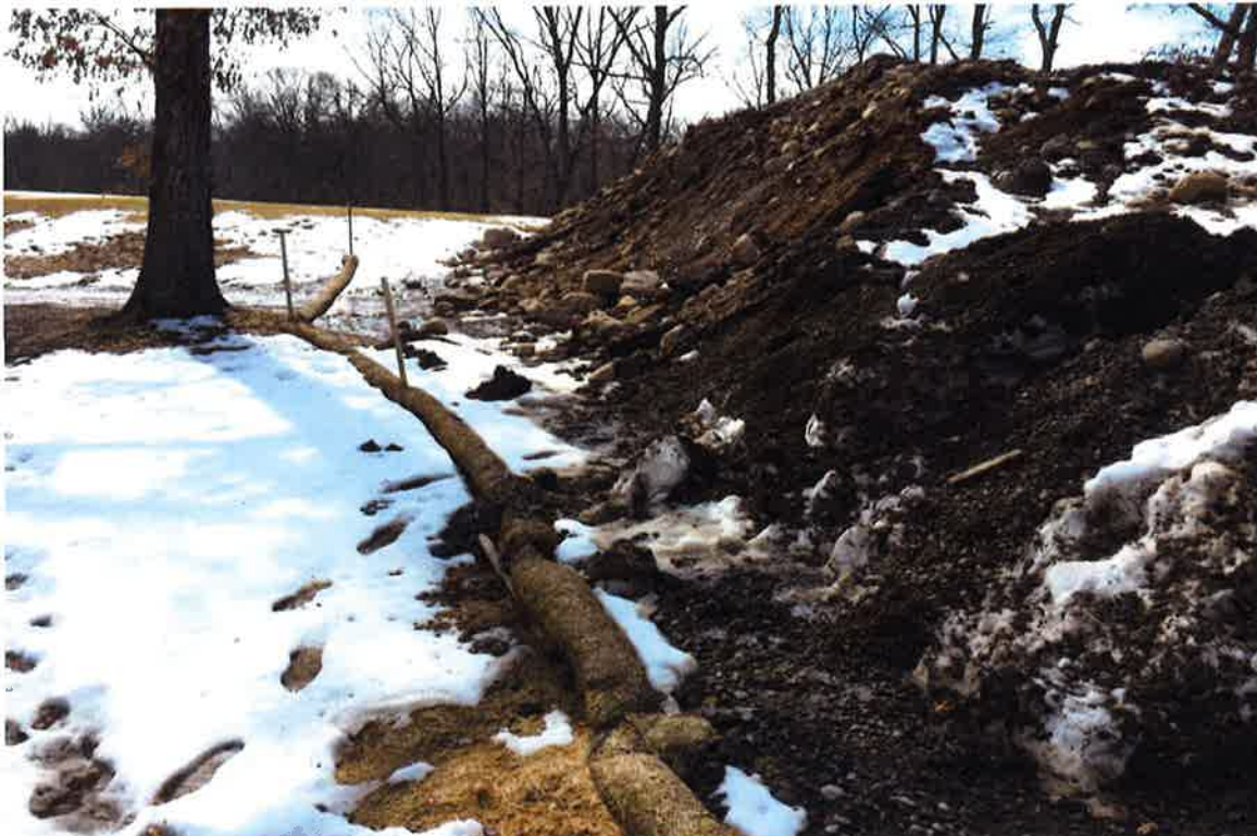
Photo 6: View of excavation storage pile.
