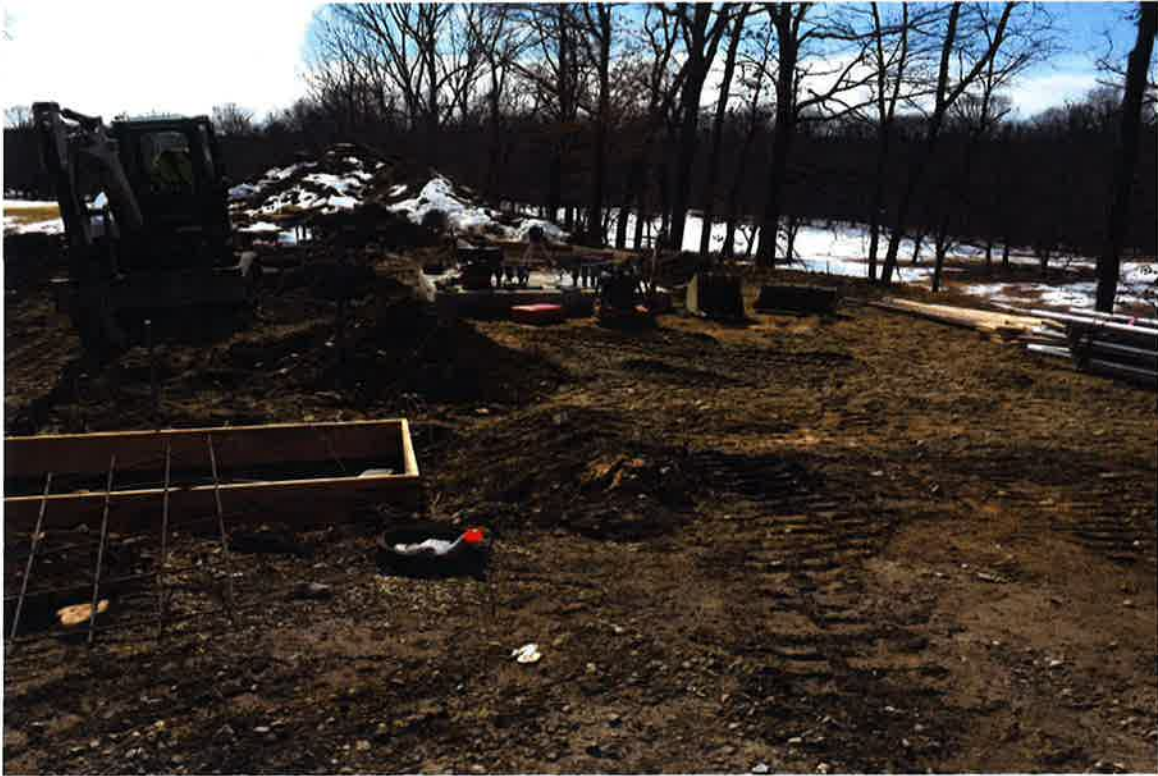
Photo 3: View of ongoing tower foundation work.
