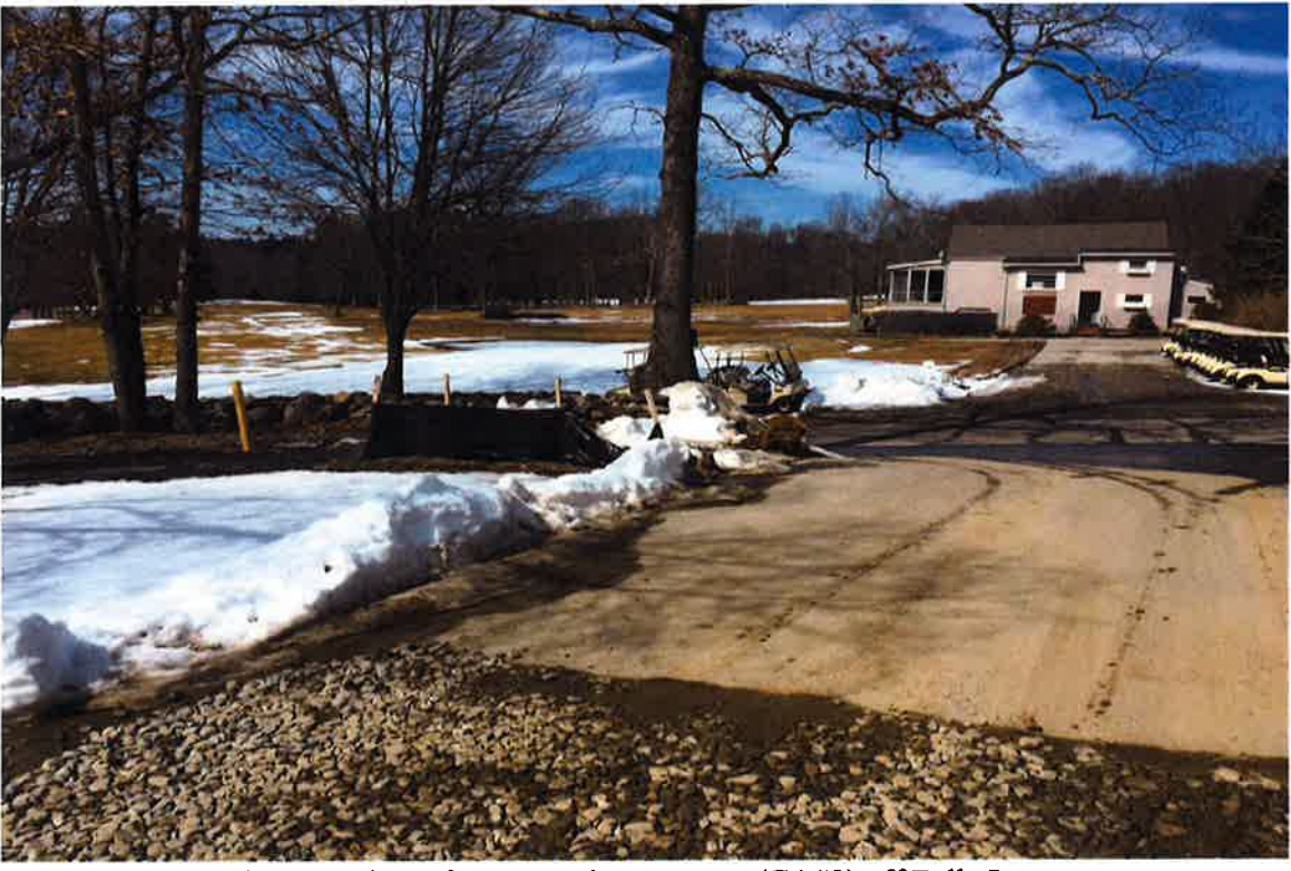
Photo 2: View of construction entrance (CA#2) off Folly Lane.
