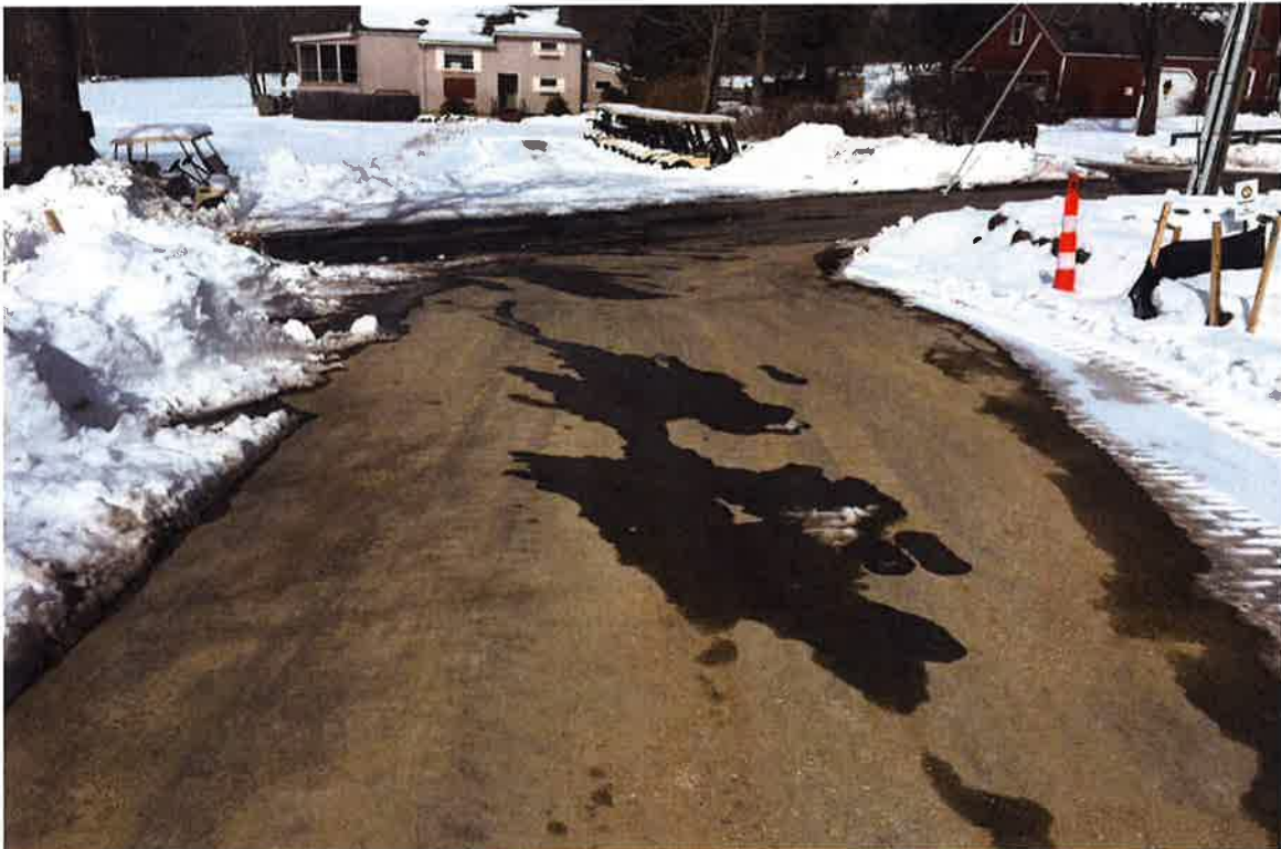
Photo 2: View of construction entrance off Folly Lane.
