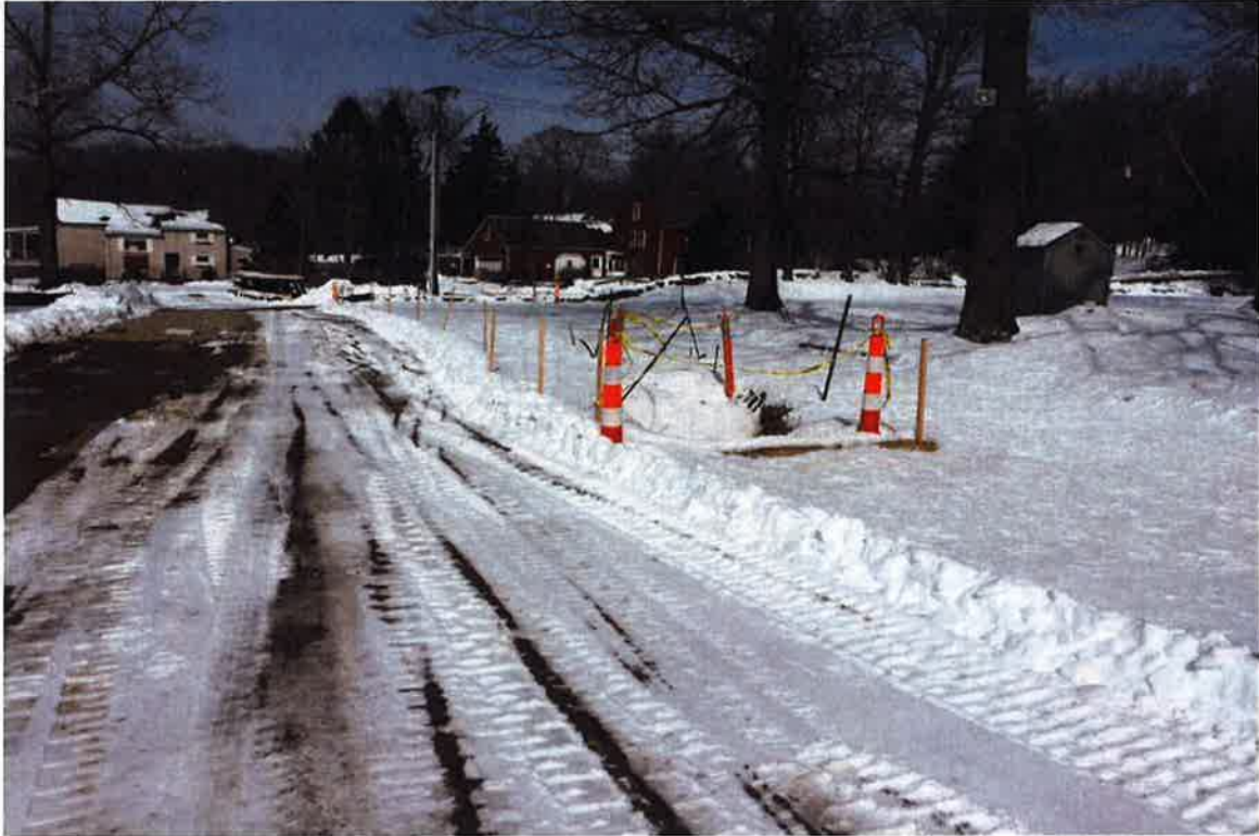
Photo 5: View of inactive utility trench work.
