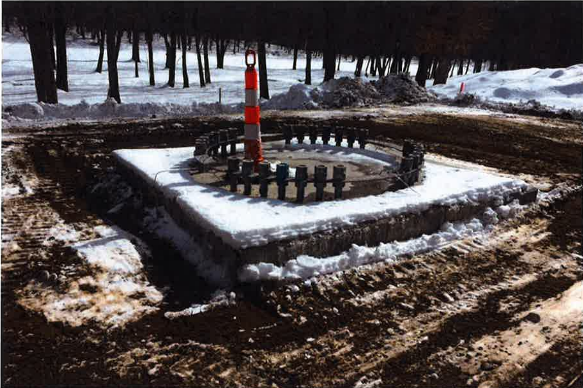
Photo 3: View of tower foundation work completed.
