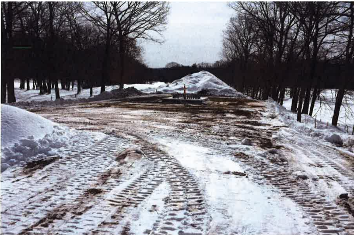
Photo 4: View of access road into compound area.
