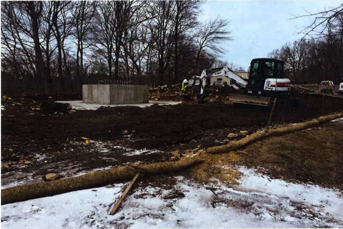
Photo 3: View of foundation work underway.
