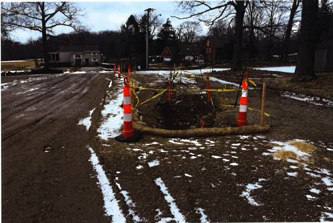
Photo 5: View of inactive utility trench work.
