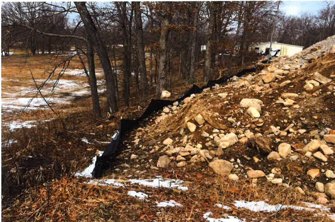
Photo 8: View of excavation material stockpile.
