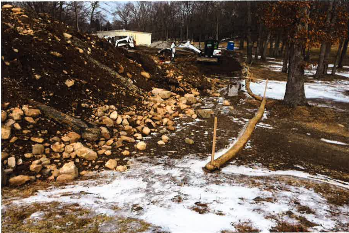
Photo 7: View of excavation material stockpile.
