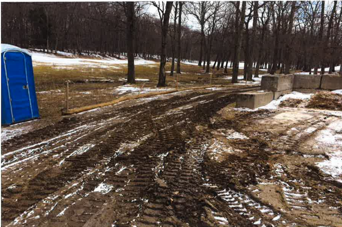
Photo 4: View of pre-existing washout location by bulk storage bins.
