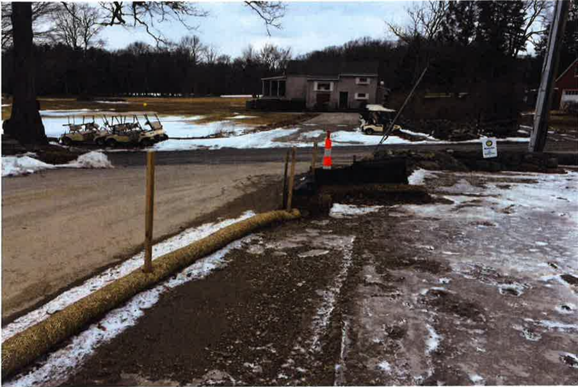
Photo 1: View of erosion controls at construction entrance off Folly Lane.
