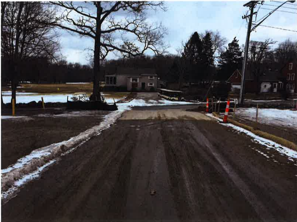
Photo 2: View of erosion controls at construction entrance off Folly Lane.
