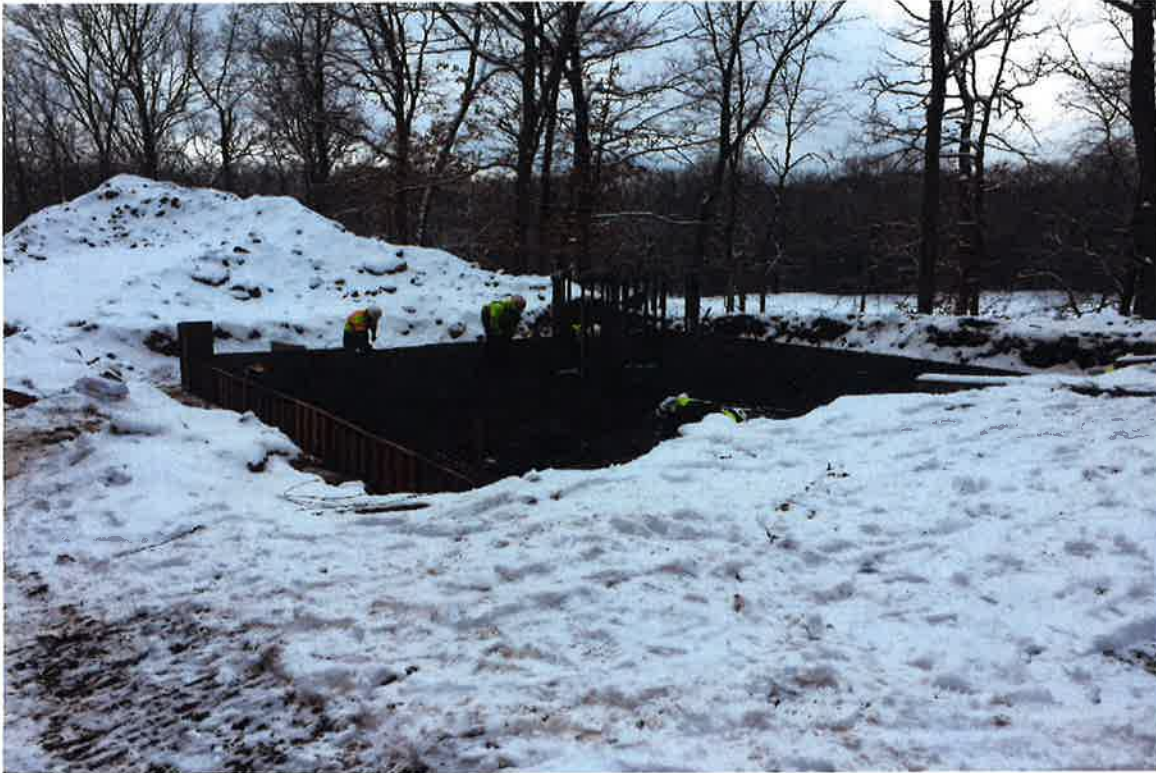
Photo 5: View of foundation work underway.
