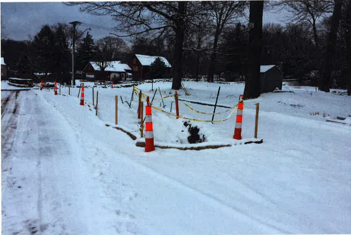
Photo 9: View of inactive utility trench.
