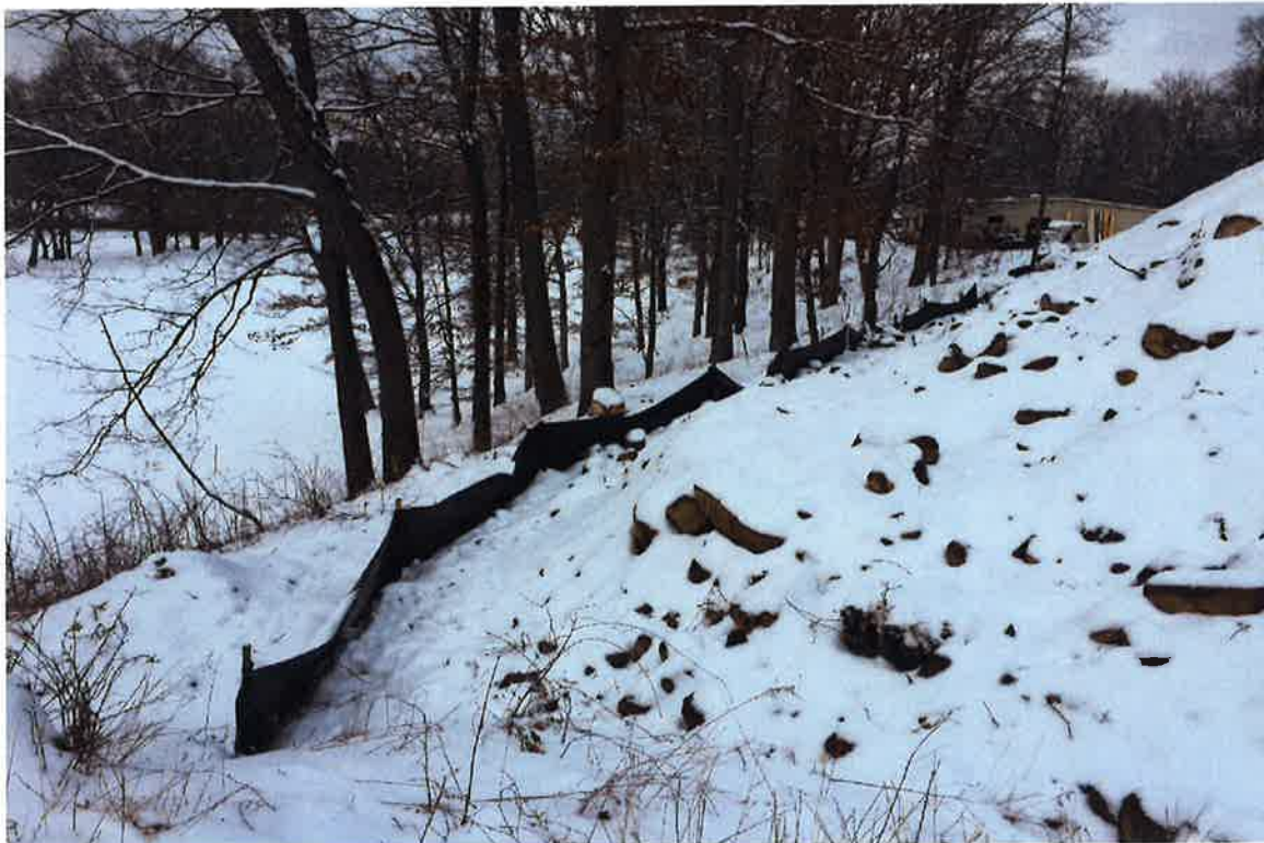
Photo 8: View of excavation material stockpile.
