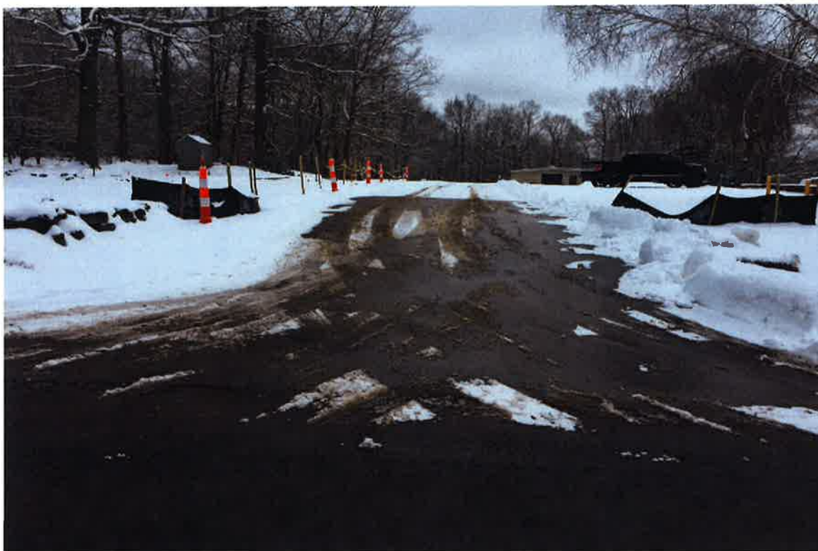
Photo 3: View of construction entrance looking from Folly Lane.
