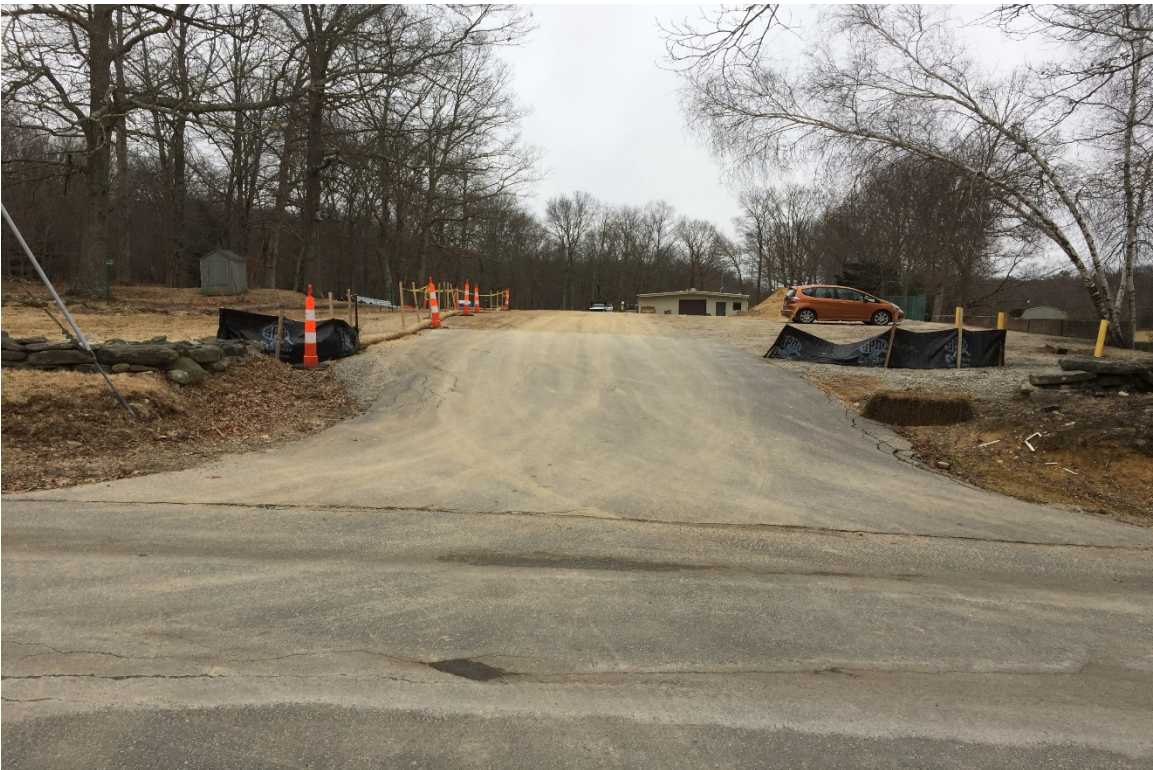
Photo 4: View of construction entrance looking towards access road to compound location.
