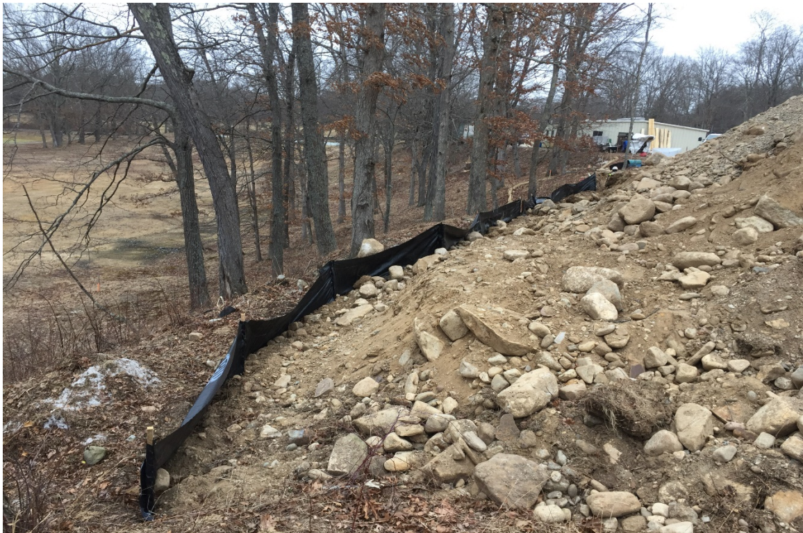
Photo 6: View of western side of excavation material storage pile.
