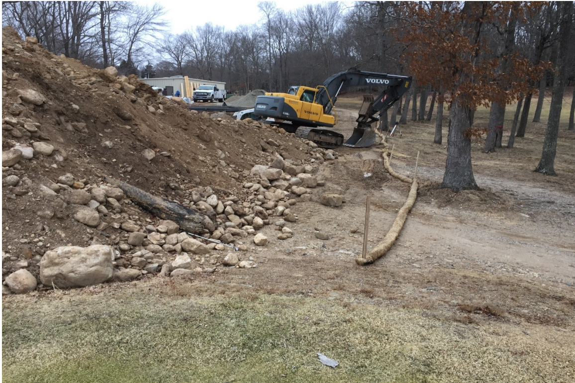
Photo 5: View of eastern side of excavation material storage pile.
