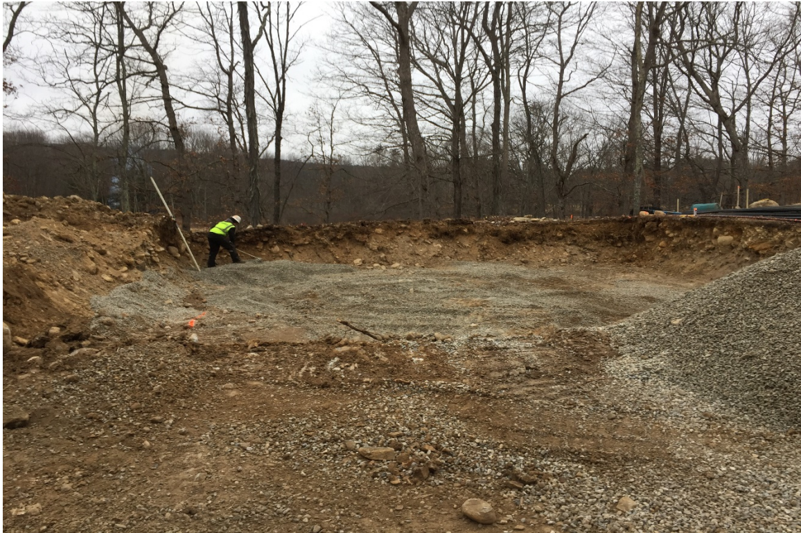
Photo 9: View of compound foundation under construction.
