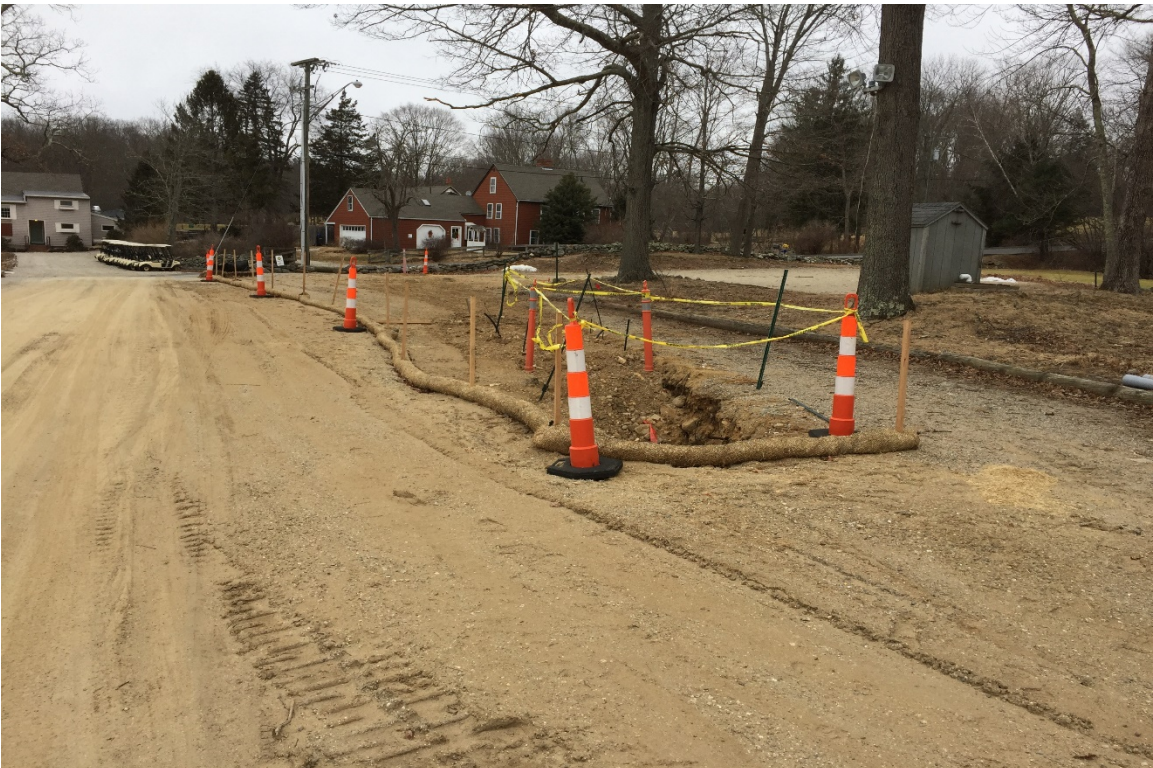
Photo 8: View of suspended utility trenching work area.
