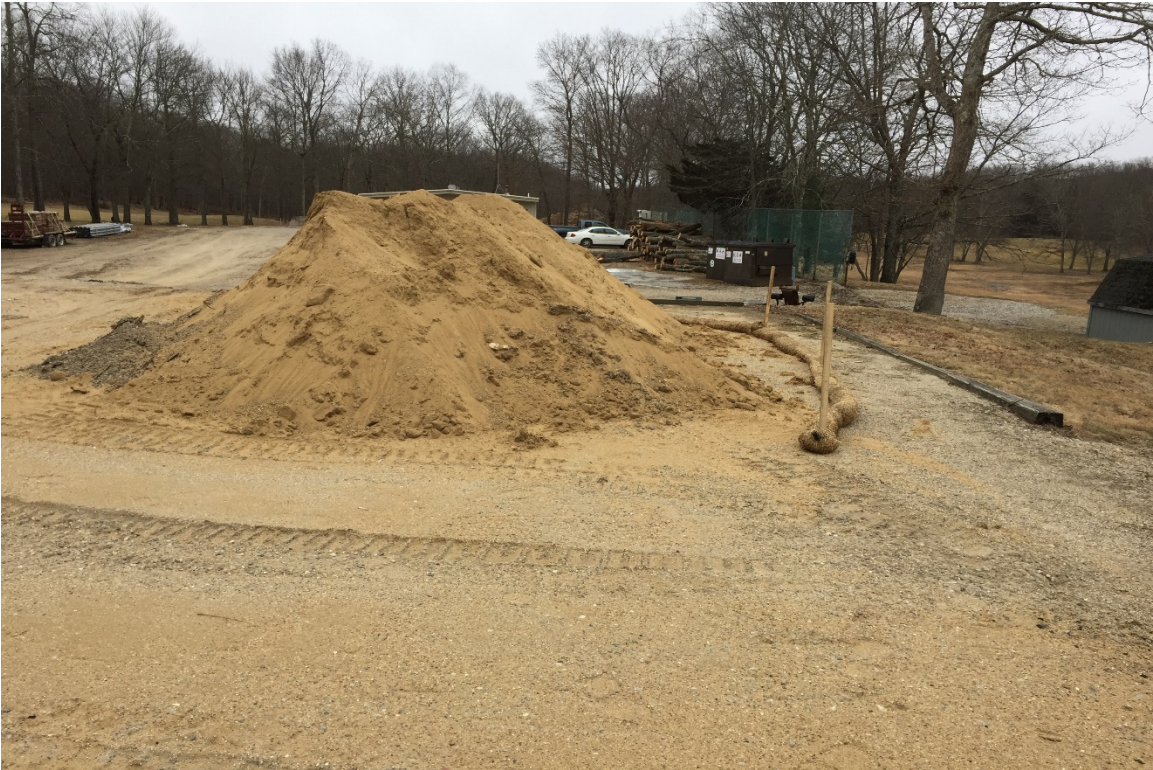
Photo 7: View of material stockpile.
