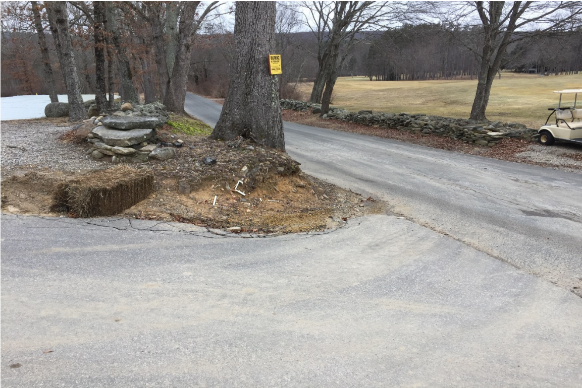
Photo 3: View of construction entrance looking towards Folly Lane.
