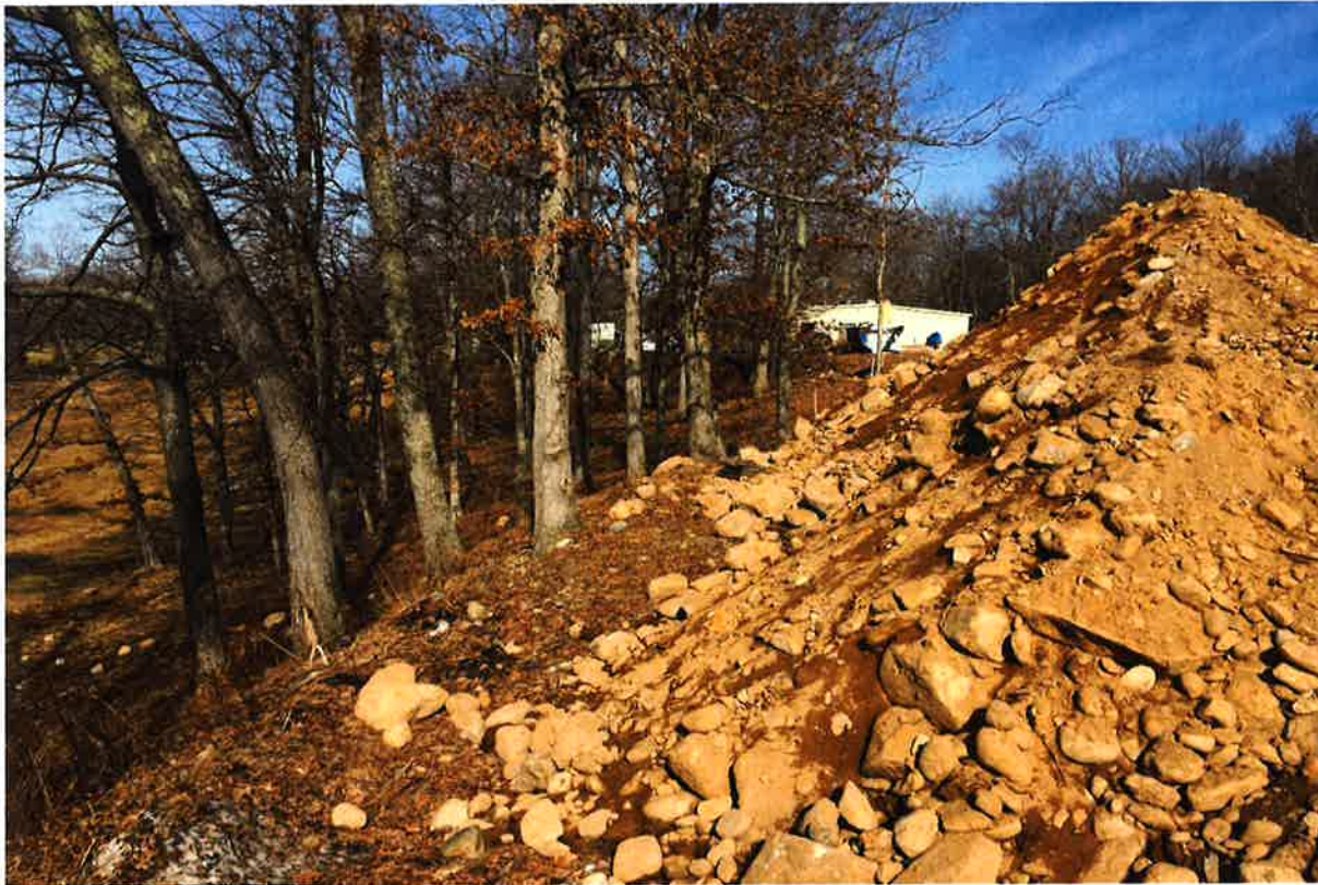
Photo 7: View of excavation material storage pile. Photo taken on February 6, 2019.
