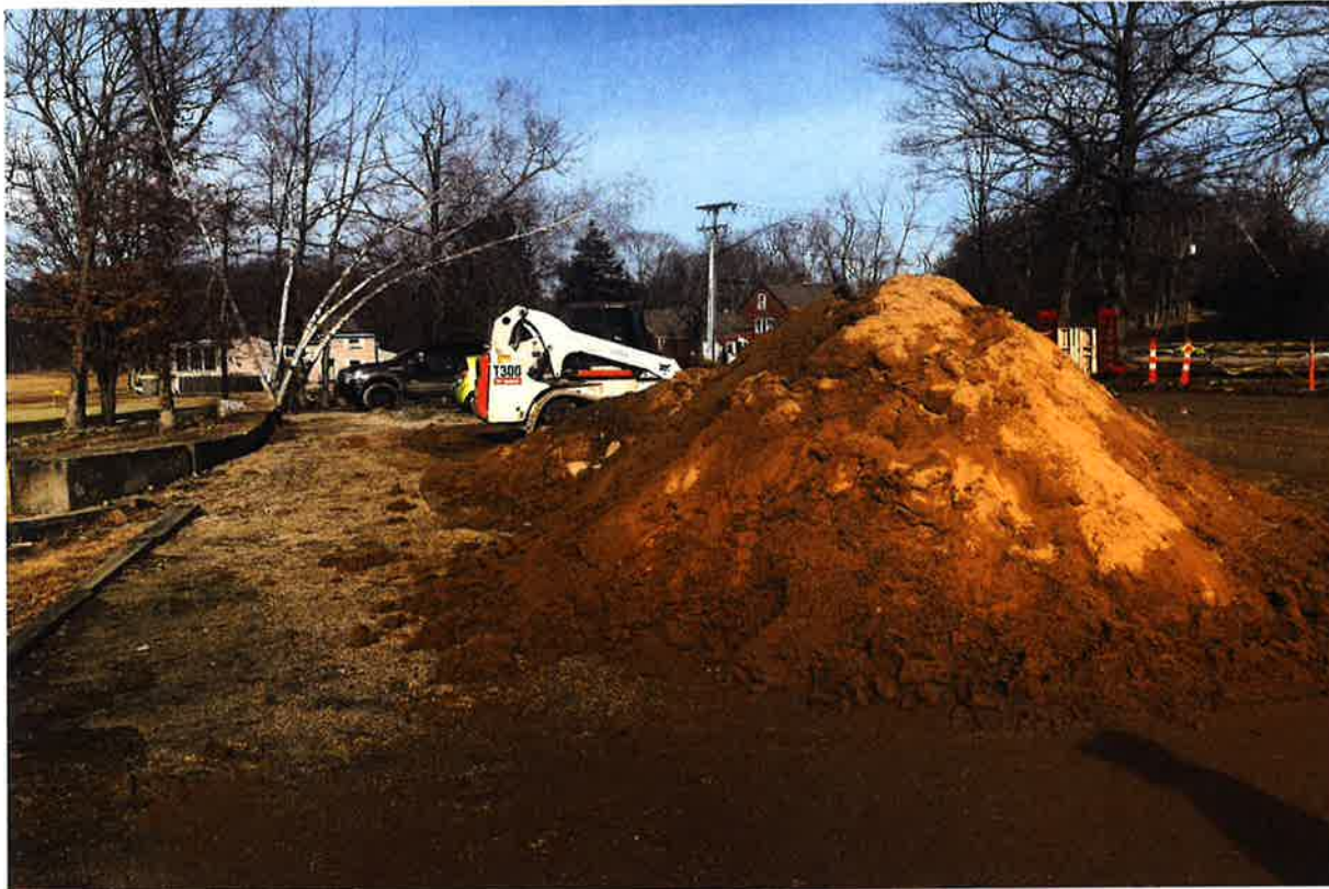
Photo 5: View of backfill stockpile. Photo taken on February 6, 2019.
