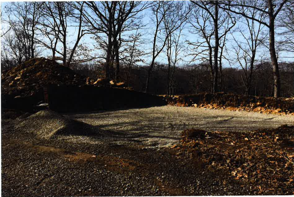
Photo 11: View of compound foundation under construction. Photo taken on February 6, 2019.
