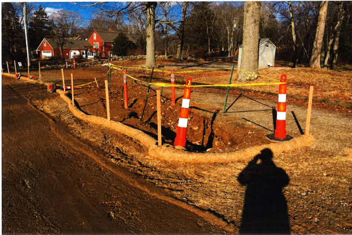
Photo 10: View of utility trenching work. Photo taken on February 8, 2019.
