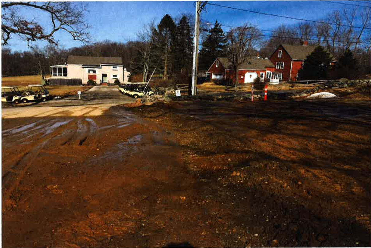
Photo 9: View of utility trenching work. Photo taken on February 6, 2019.
