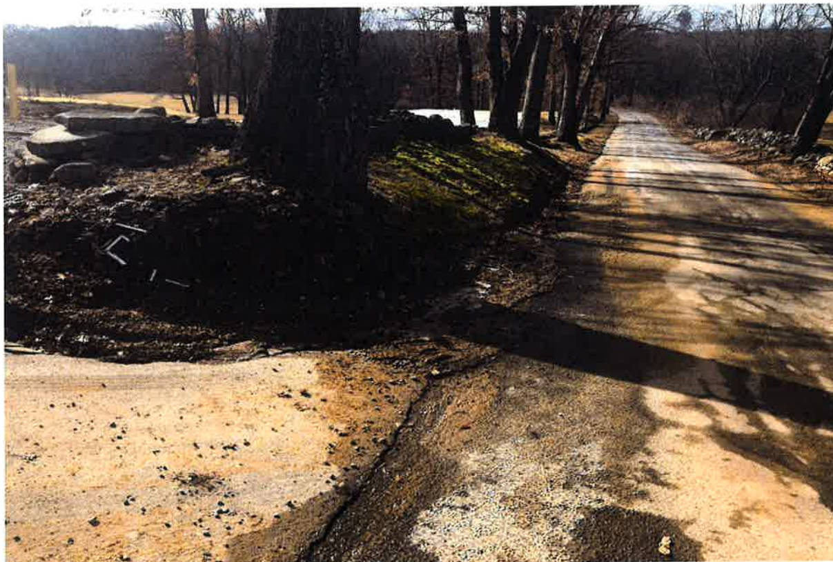
Photo 1: View of pre-existing washout at Folly Lane entrance. Photo taken on February 6, 2019.
