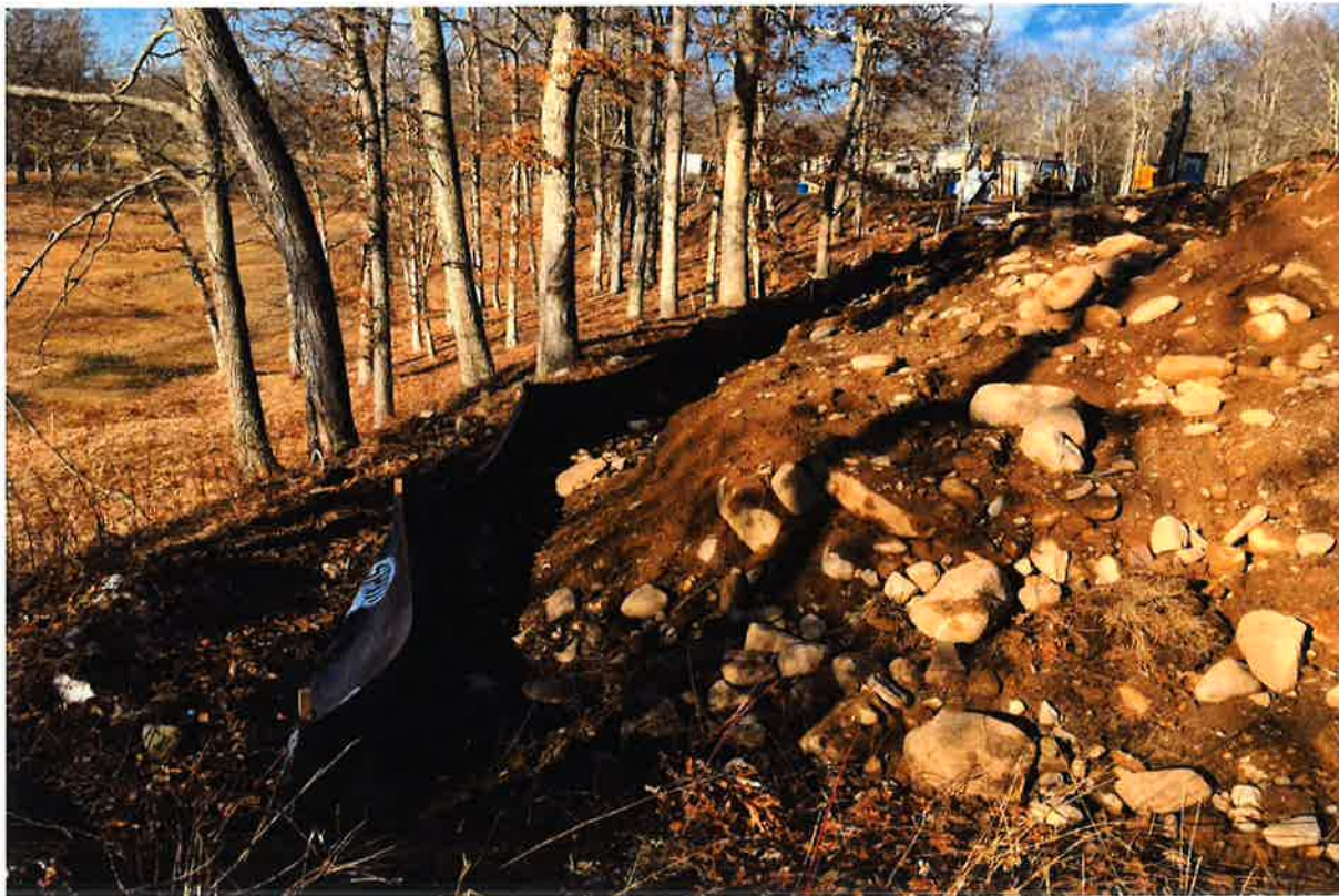
Photo 8: View of excavation material storage pile. Photo taken on February 8, 2019.
