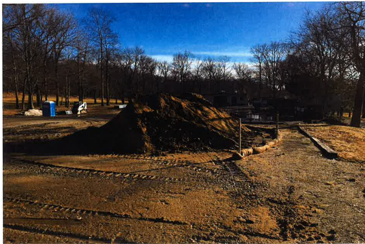
Photo 6: View of backfill stockpile. Photo taken on February 8, 2019.
