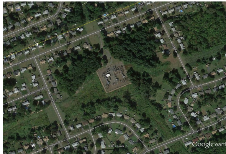
Newington Substation (access off of Cherry Hill Drive, Newington)
