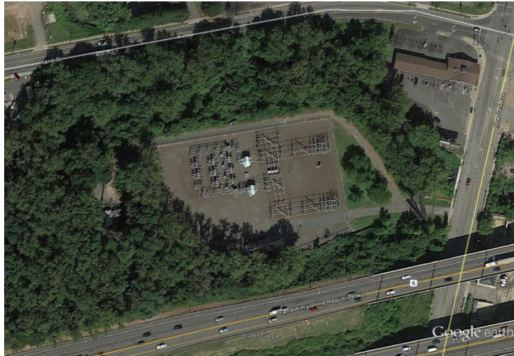
Southwest Hartford Substation (access off of New Park Avenue, Hartford)
