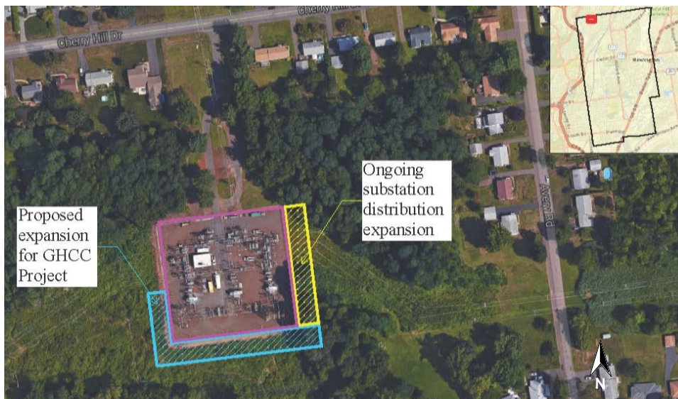
Aerial of Newington Substation (access off of Cherry Hill Drive, Newington)
