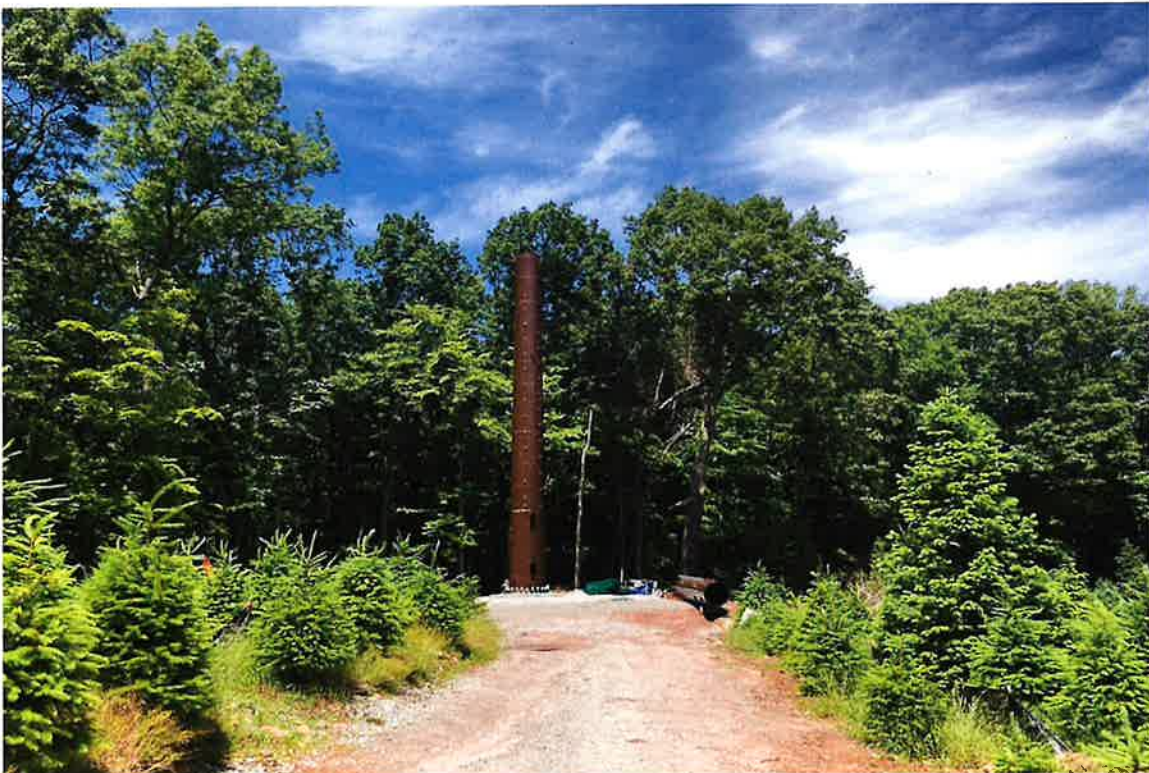
Photo 2: View of first section of tower erected.
