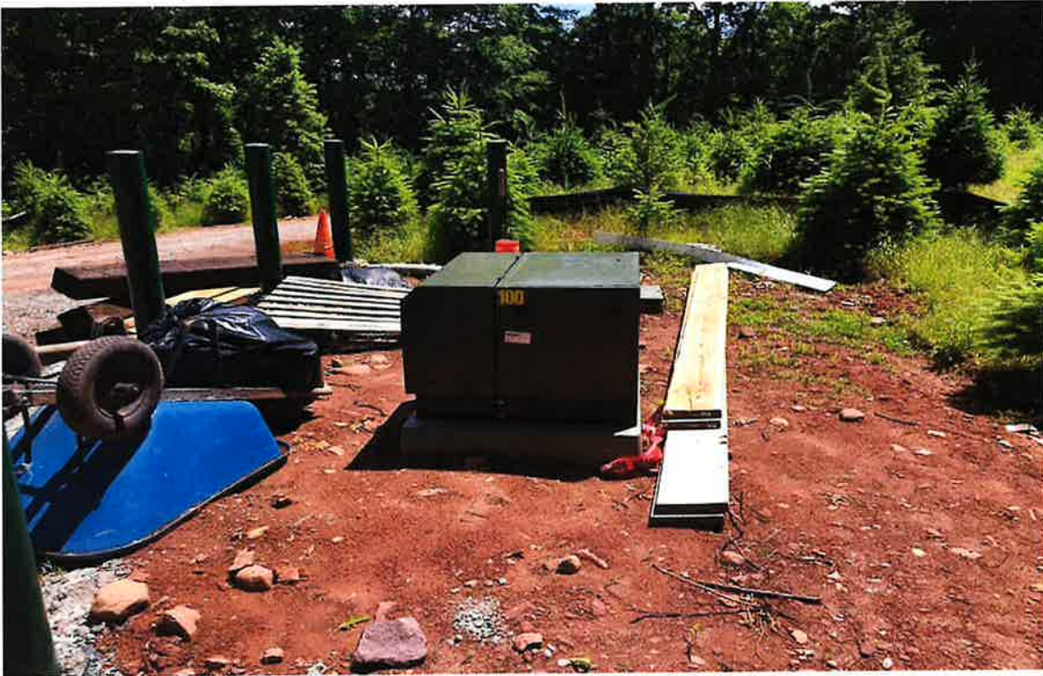
Photo 5: View of completed utility work.
