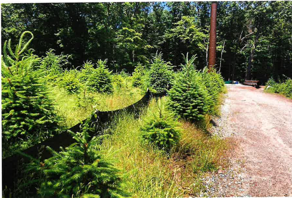
Photo 4: View of silt fence maintained.
