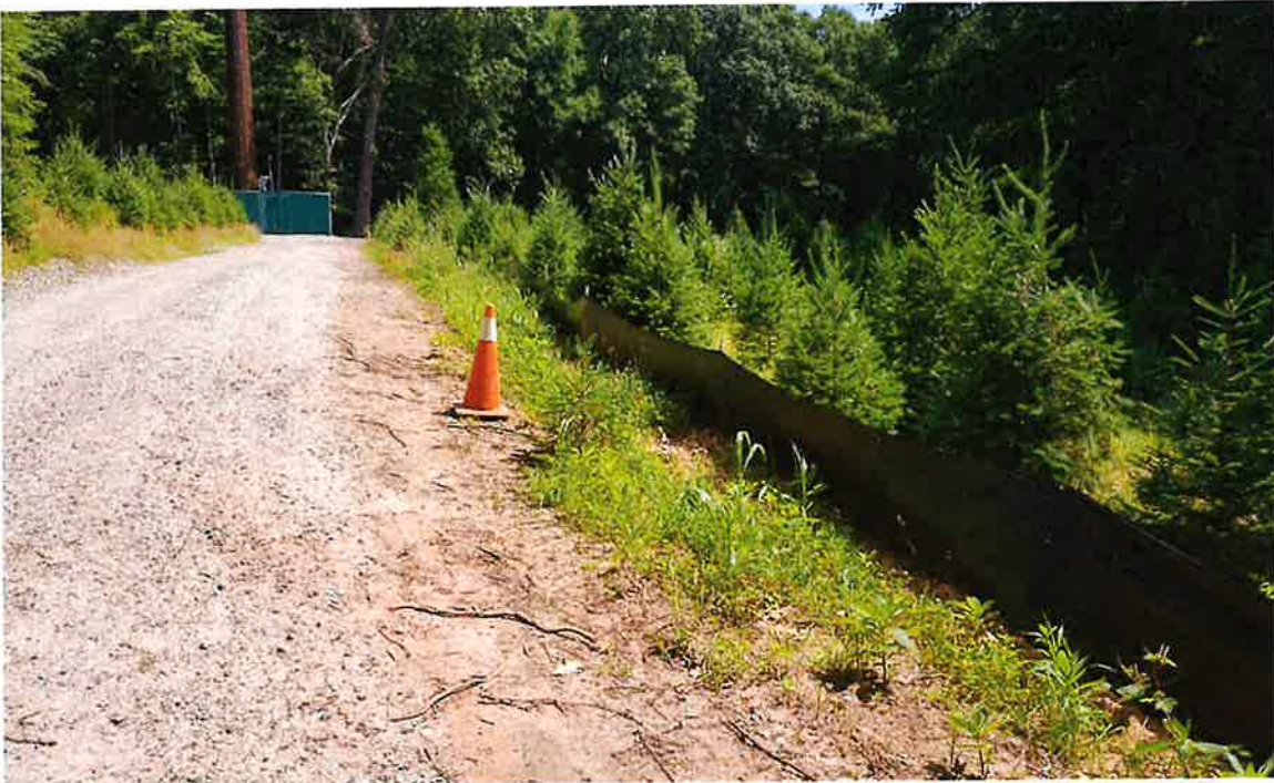
Photo 3: View of properly installed/maintained exclusionary silt fence.
