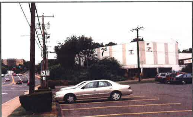
Vacant 7 th Ave. Building
