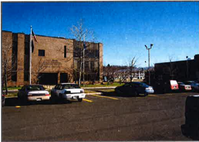
East Shore Water Pollution Treatment Facility
