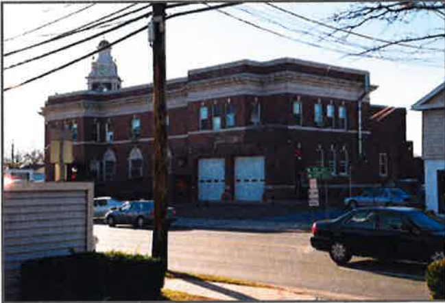
Hamden Fire Department - Dixwell Avenue Station
