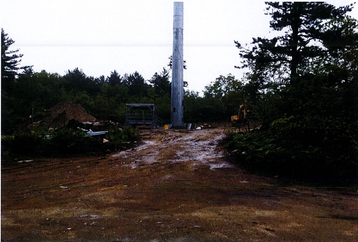
Photo 2: View of compound under construction looking north.
