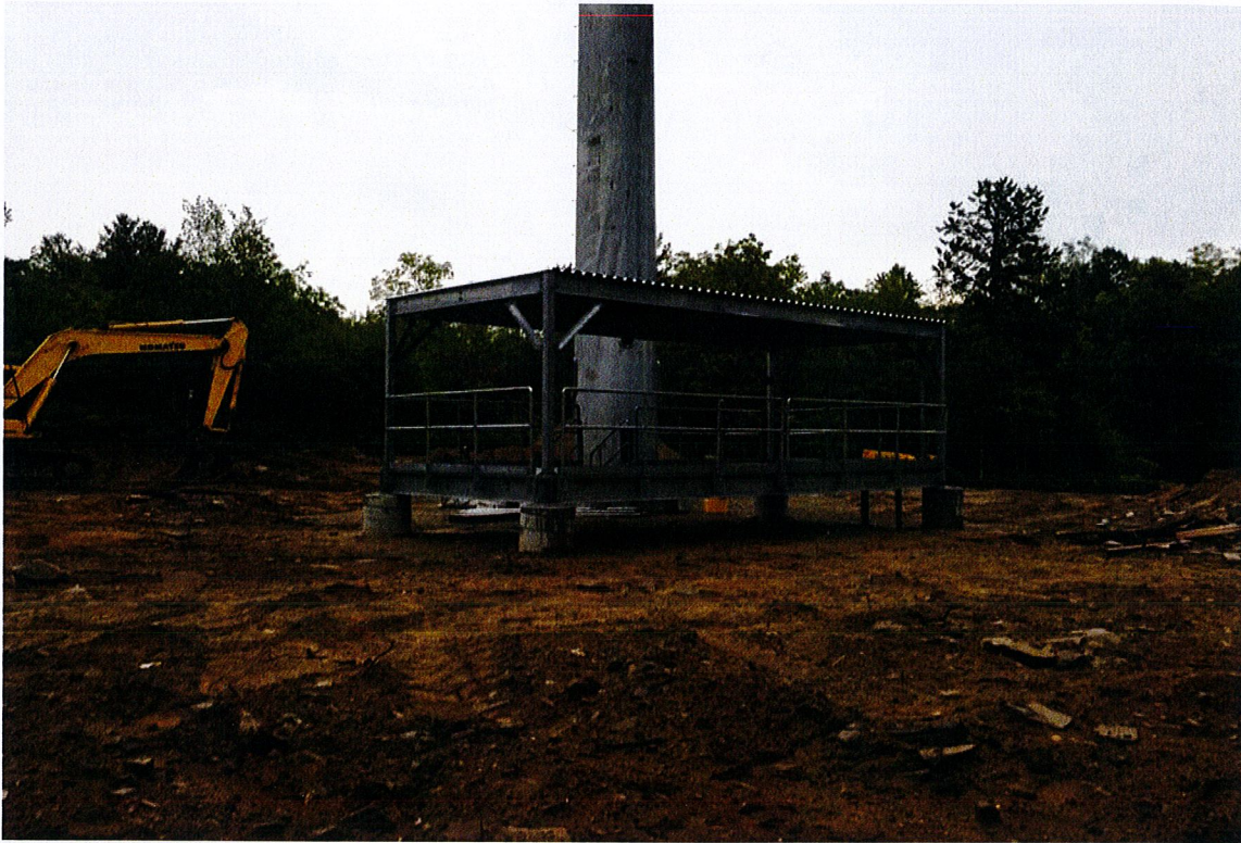
Photo 3: View of compound under construction looking east.
