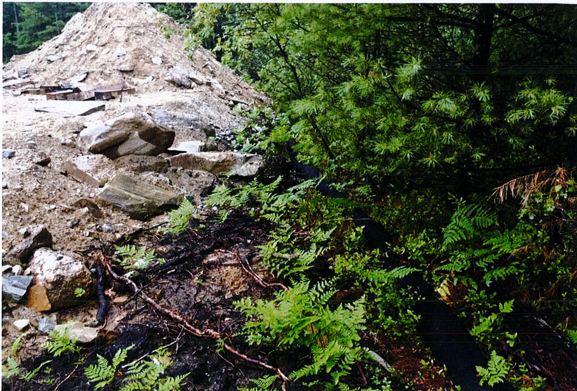
Photo 4: View of compost filter sock looking south.
