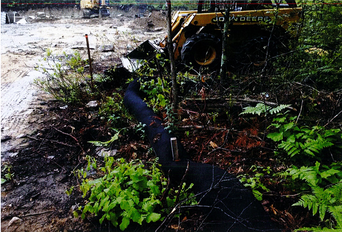
Photo 5: View of compost filter sock surroundings site.
