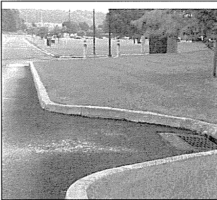
Road with Stormwater Management
