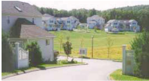
Preserved green space over the community septic leaching field at Newtown's Riverview Condominium
