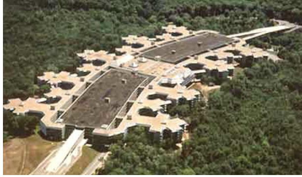
The 1.3 million square foot Corporate Center in Danbury is the largest office building in Connecticut.
