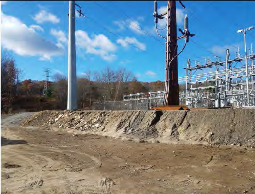
Photo 10: 11/17/2017, Watertown: Map 01, Str1A, rill erosion and sedimentation down gradient of work pad.
