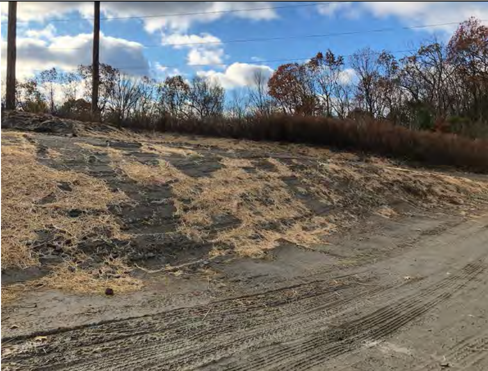
Photo 9: 11/17/2017, Watertown: Map 02, Str4, windblown straw covering seed on slope and top of pad.
