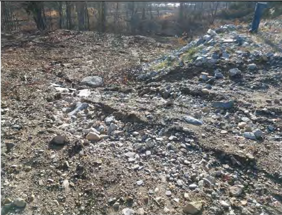
Photo 11: 11/17/2017, Watertown: Map 01, down gradient of Str1A, rill erosion and sedimentation down gradient to the east toward the Connecticut Wetland Only designated area.
