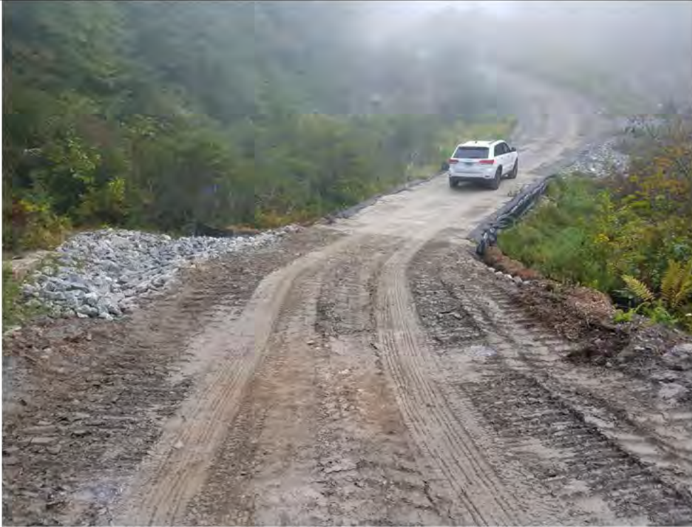
Photo 1: 09/15/17, Watertown: Map 14, access road north of Str39 to wetland W-C20, water bar flattened out. No changes in road conditions from previous inspection on 09/08/15.
