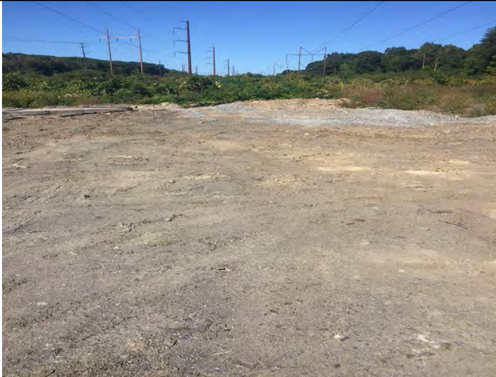
Photo 12: UPDATE provided on 09/27/17, Information and photo received from Matt Davison of Davison Environmental. The petroleum release area observed at Str15 and Str14 (Map 6) was reported on 09/22/2017 to the CTDEEP (spill #201704861, badge #205) and removal of the impacted pad material was completed.
