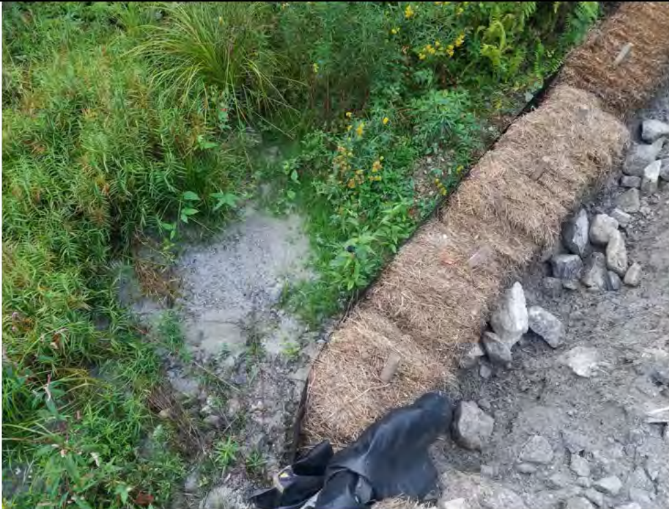
Photo 3: 09/15/17, Watertown: Map 14, at southeast corner of timber mat crossing over wetland W-C20, breakthrough into W-C20, photo taken at the time of this inspection. SEE PHOTO 4 FOR CORRECTIVE ACTION following inspection.
