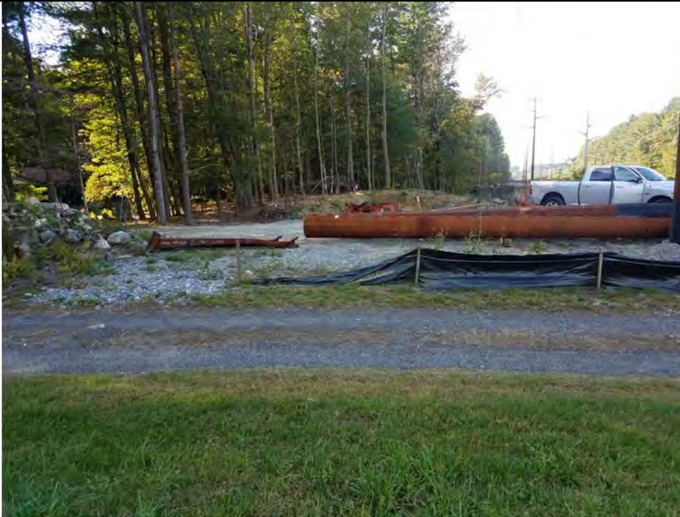
Photo 11: 09/22/17, Harwinton: Map 34, exclusion fencing along the north edge of the pad at Str94 is in need of repair/replacement.
