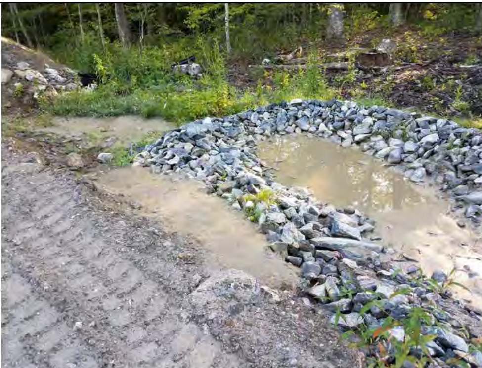
Photo 6: 09/08/2017, Watertown: Map 13, south of Str36, excess sediments in temporary basin, sediment runoff from uncontrolled storm water flow off the access road.
