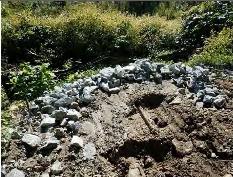
Photo 8: 09/08/2017, Watertown: Map 10, between Str26 and Str27, excess buildup of sediment in temporary sediment pond.
