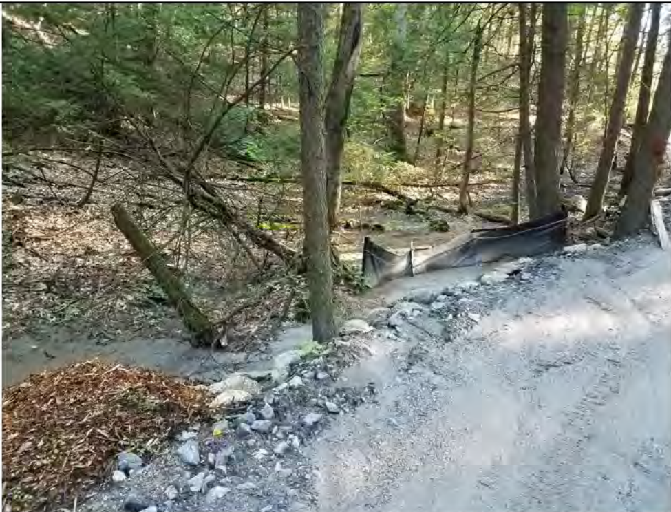
Photo 20: 09/08/2017, Watertown: Map 15, access road between Str44 and Str45 approximately 100 feet north of the CT State marked Hiking trail, rills and sediment flow off access road.
