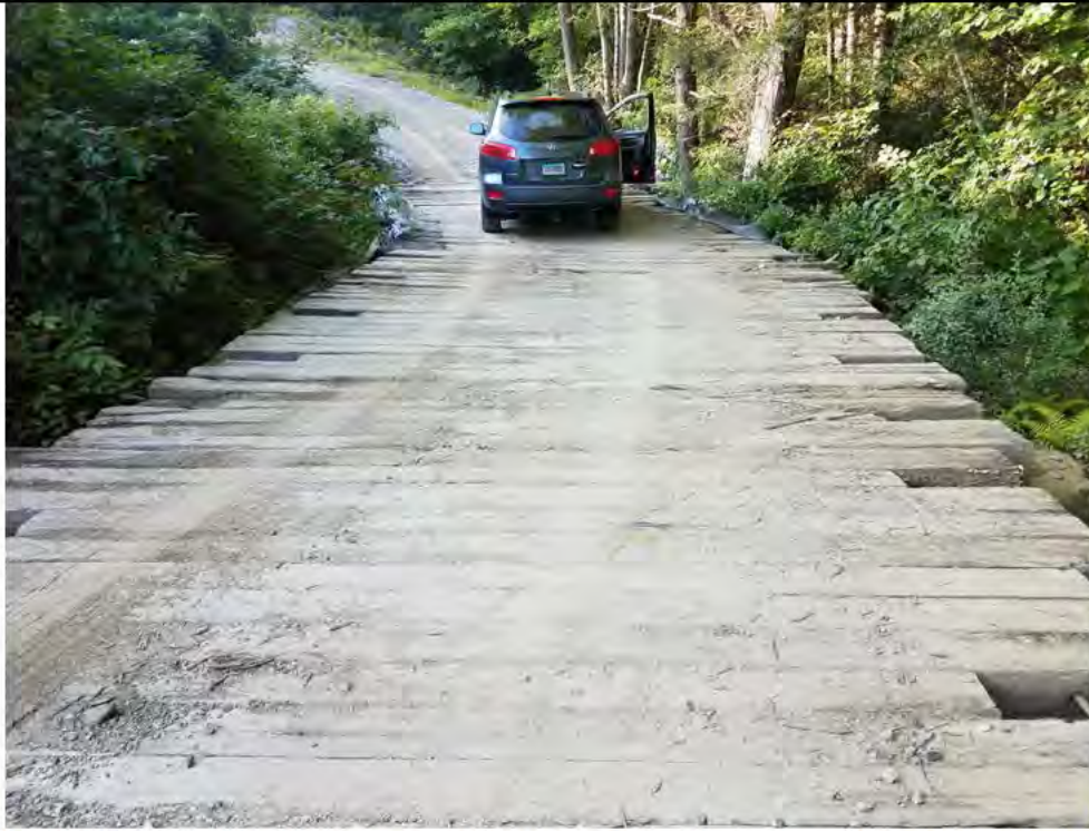
Photo 1: 09/01/2017, Watertown: Map 12, timber mat crossing at W-C15/S-C5, timbers pushed to the outside of the bend (seen at below the parked vehicle).
