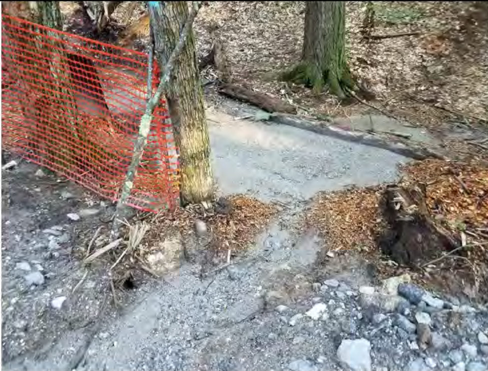
Photo 19: 09/08/2017, Watertown: Map 15, access road between Str44 and Str45 at the CT State marked Hiking trail, rills and sediment flow off access road into the access point of hiking trail.
