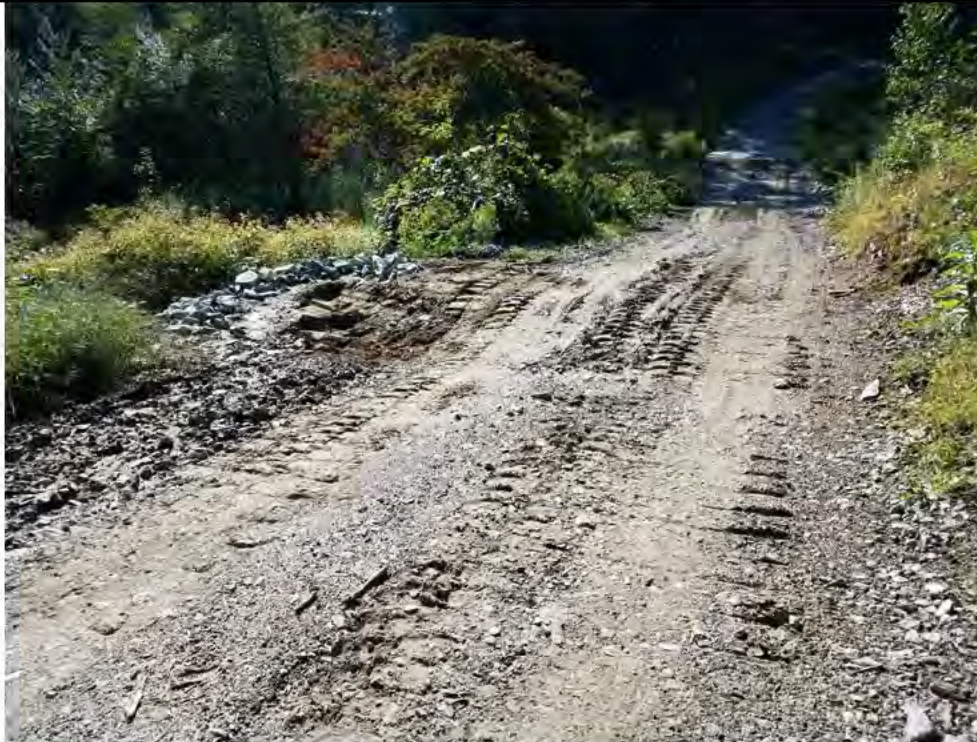
Photo 7: 09/08/2017, Watertown: Map 10, between Str26 and Str27, water bar flattened out, sediment buildup in temporary sediment pond.
