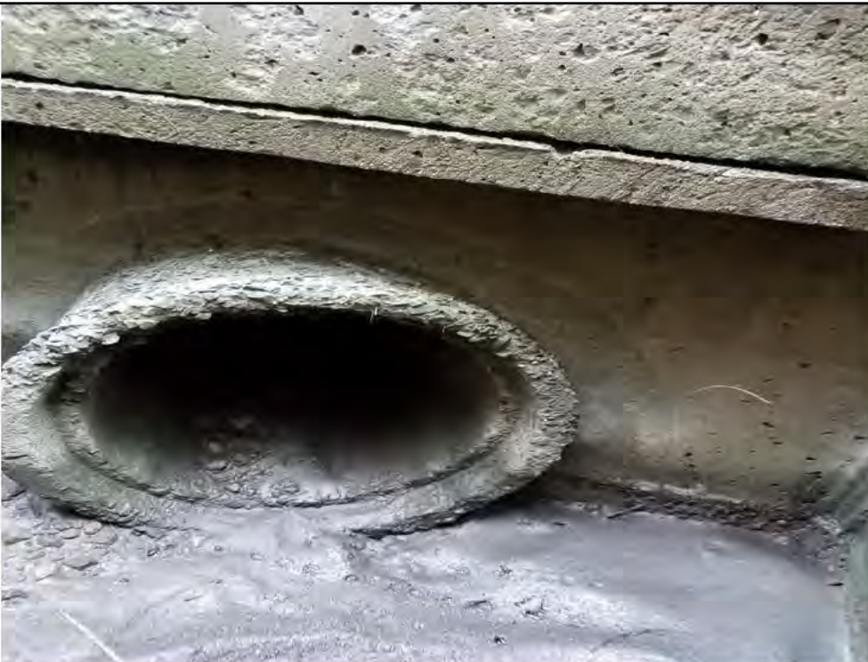
Photo 22: 09/08/2017, Litchfield, Map 29: At Str81, sediment flow into the catch basin located on Campville Road, no silt sack or catch basin protection
