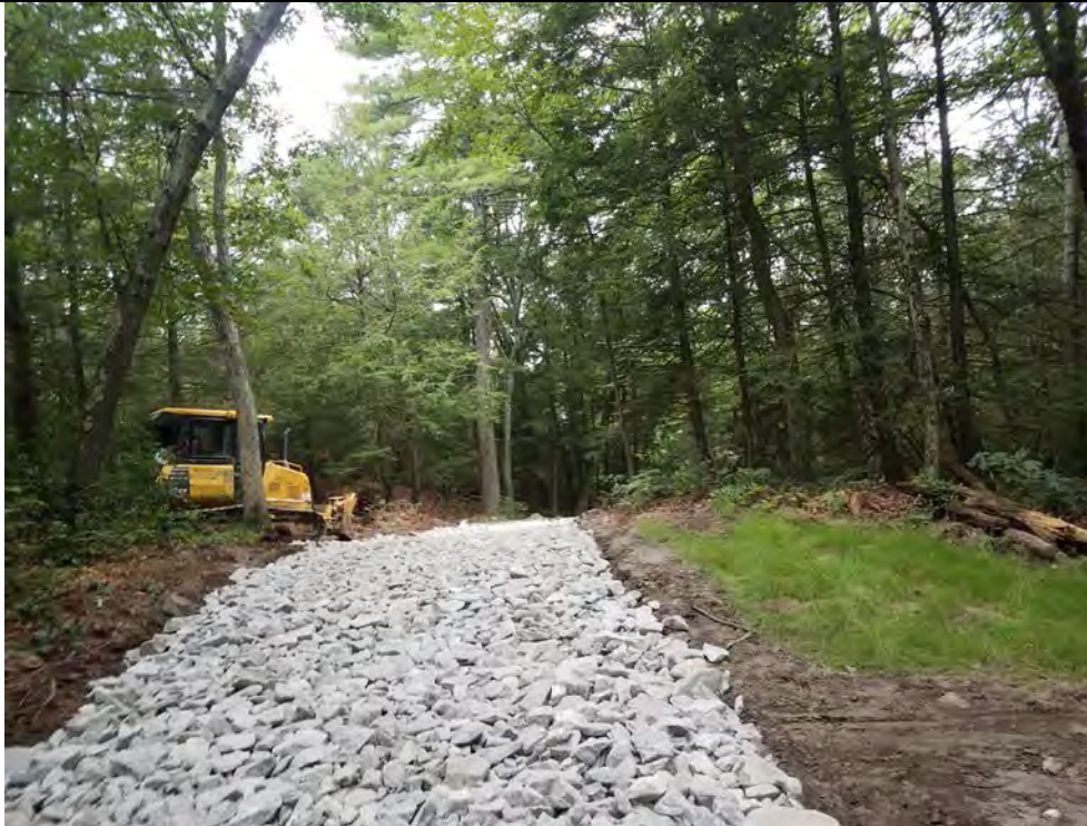
Photo 2: 08/04/2017, Watertown: Maps 14 & 15, access road improvements between Str41 and Str42.
