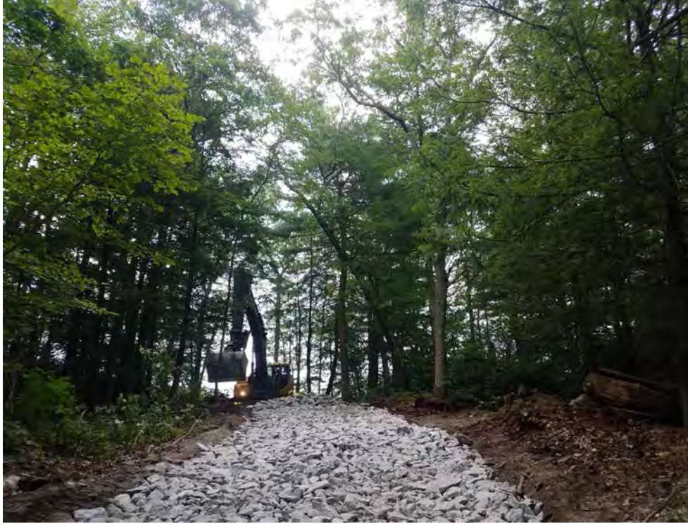
Photo 1: 08/04/2017, Watertown: Maps 14 & 15, access road improvements between Str41 and Str42.
