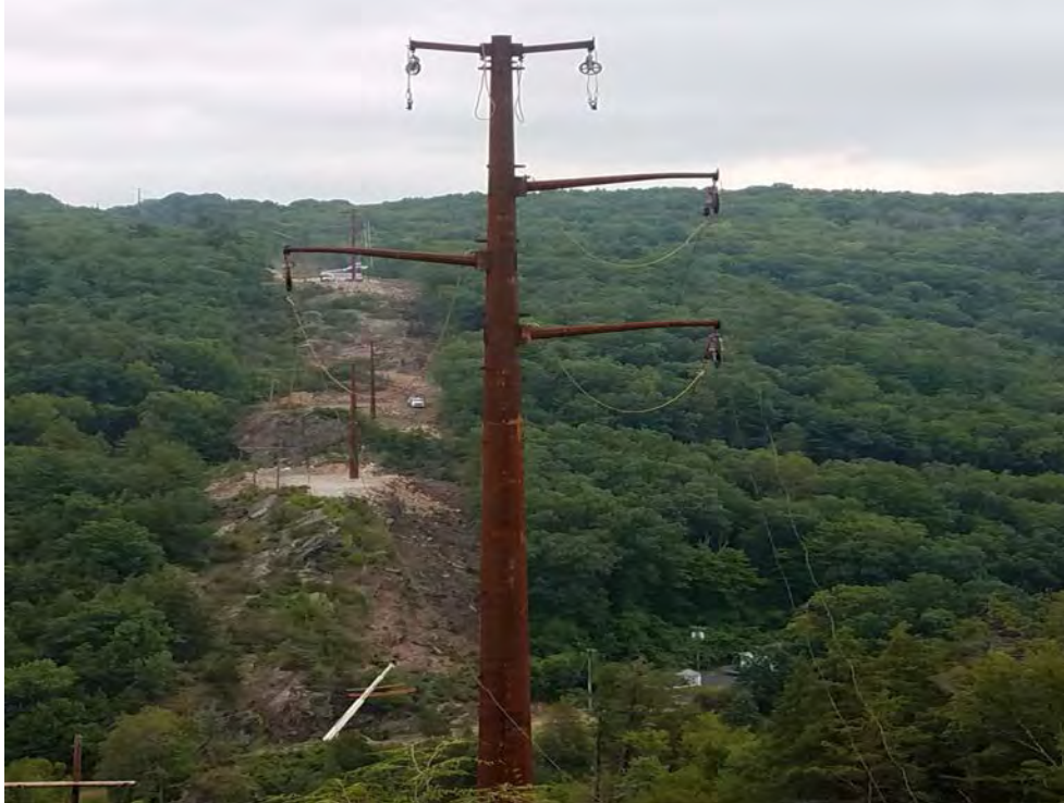
Photo 4: 08/04/2017, Watertown: Maps 16 & 17, PAR pulling cable from Str47 through Str46 to Str45.
