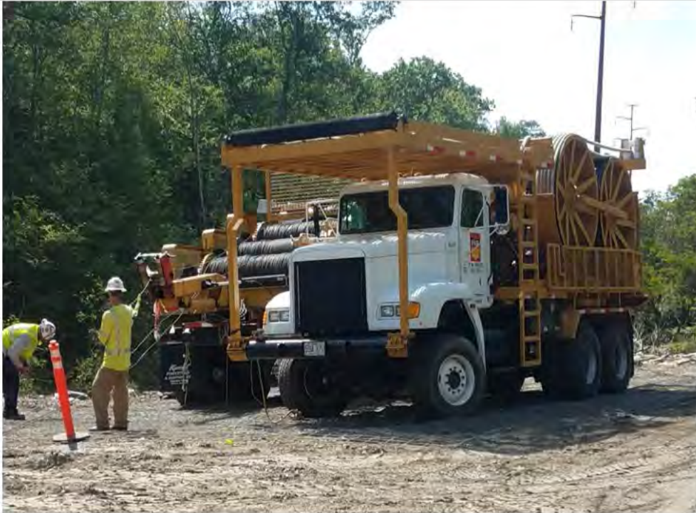
Photo 6: 08/11/17: Watertown, Map 14, Str39, and PAR setting up to pulling cable.
