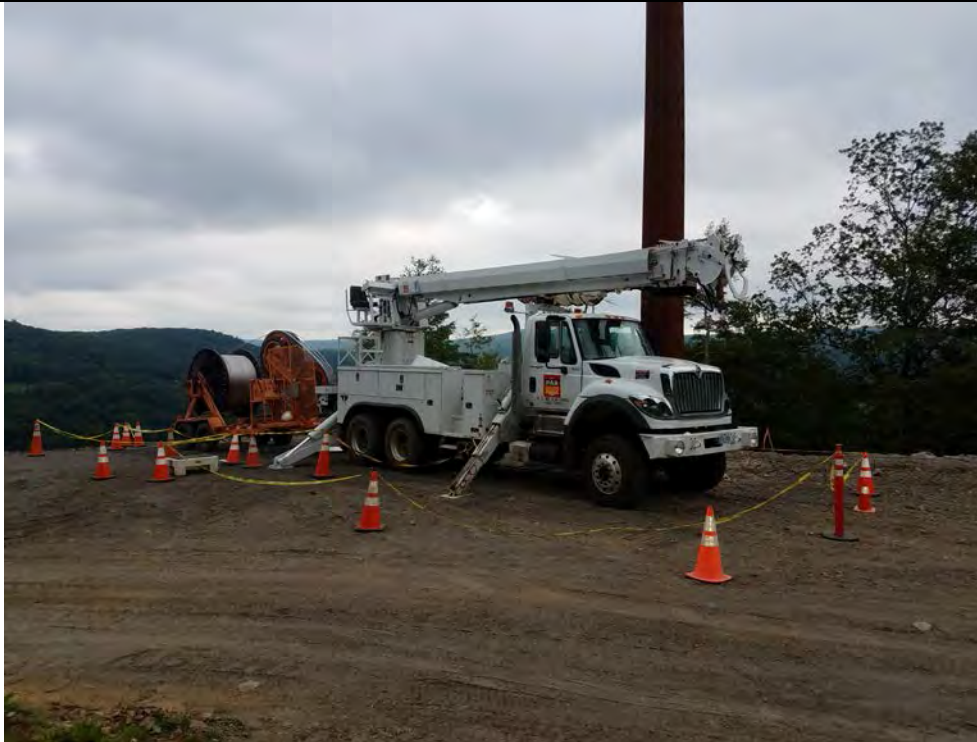
Photo 3: 08/04/2017, Watertown: Map 16, PAR set up to pull cable to Str45.
