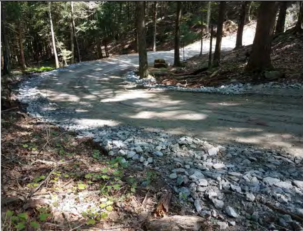
Photo 8: 08/11/17: Watertown, Map 15, finished access road construction (New) between Str42 and Str43.
