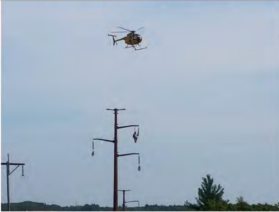
Photo 5: 08/11/17: Watertown, Map 14, Str41, and PAR setting pulleys with helicopter.
