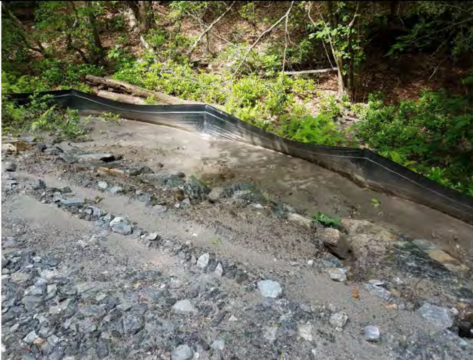
Photo 2: 06/23/2017, Watertown: Map 15, access road between Str41 and Str42, Silt fence maintenance required (Along the same silt fence line as Photo 1 above). UPDATE-As of 6/27/2017, Matt Davison reported this area is being worked on.
