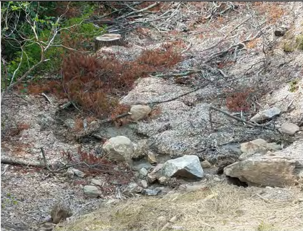
Photo 4: 06/23/2017, Watertown: Map 15, Str42 pad, At south end of the pad, storm water runoff is channeled to the slope via cut swale and fine sediments from the pad materials are travelling down the slope to the south. UPDATE-As of 6/27/2017, Matt Davison reported that this area is being worked on.
