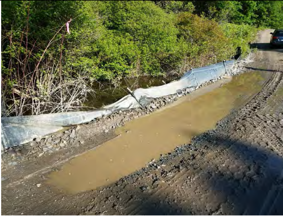
Photo 1: 06/02/2017, Watertown: Map 10, E&S control maintenance and access road improvements required at wetland W-C3.
