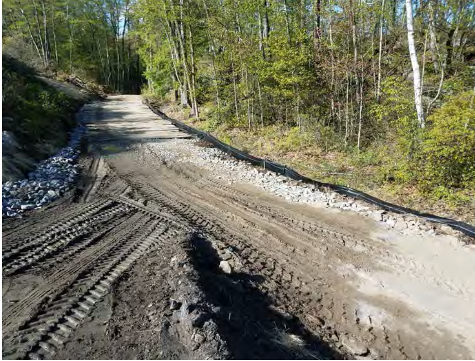
Photo 1: 05/12/2017, Watertown: Map 13, E&S (Silt Fence) controls repaired.
