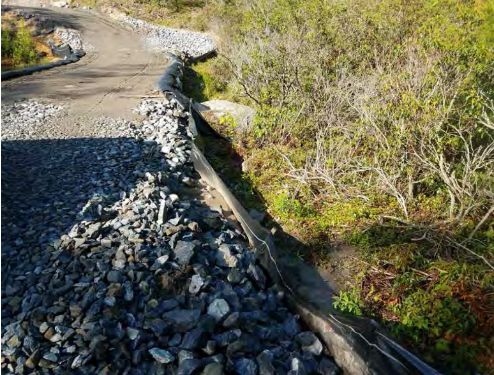
Photo 7: 05/19/2017, Watertown: Map 14, timber mat crossing at VP-C20-1 in need of cleaning and maintenance of perimeter silt fence.
