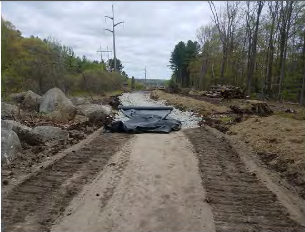
Photo 4: 05/12/2017, Litchfield: Map 28, Access road construction between Str79 and Str80.
