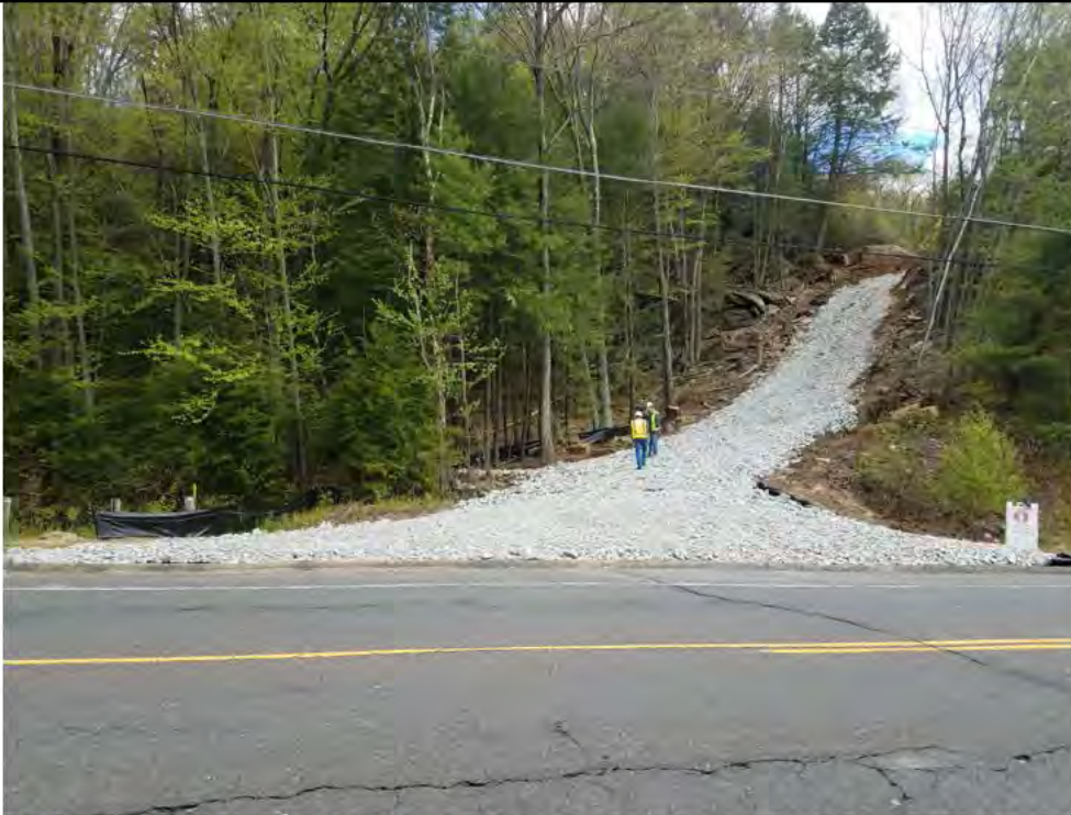
Photo 3: 05/12/2017, Thomaston: Map 17, tracking pad/apron and access road construction at Str48.
