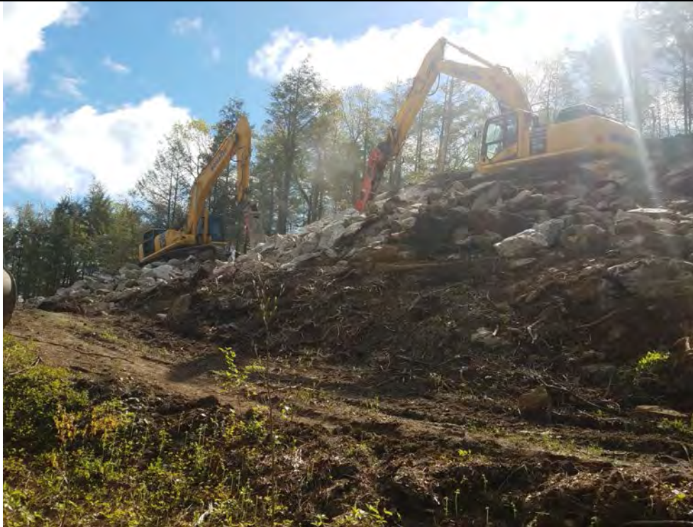
Photo 2: 05/12/2017, Watertown: Map 15, Rock Hammering pad at Str44.
