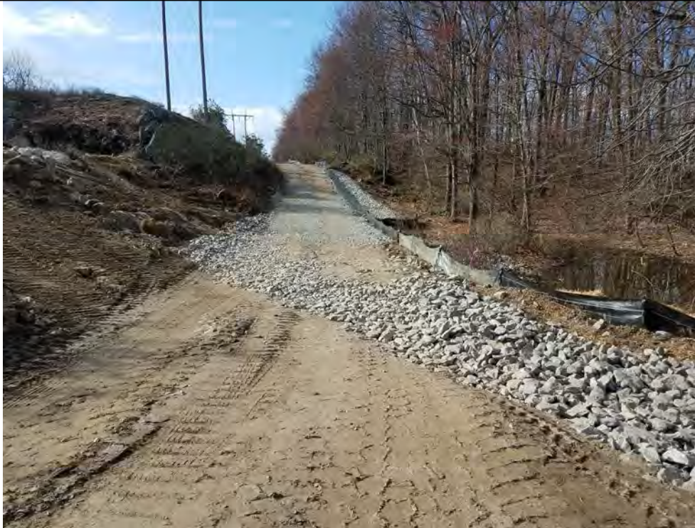
Photo 7: 4/14/2017, Watertown: Map 11, access road, water bar, stone swale and E&S improvements in the area of Str31.
