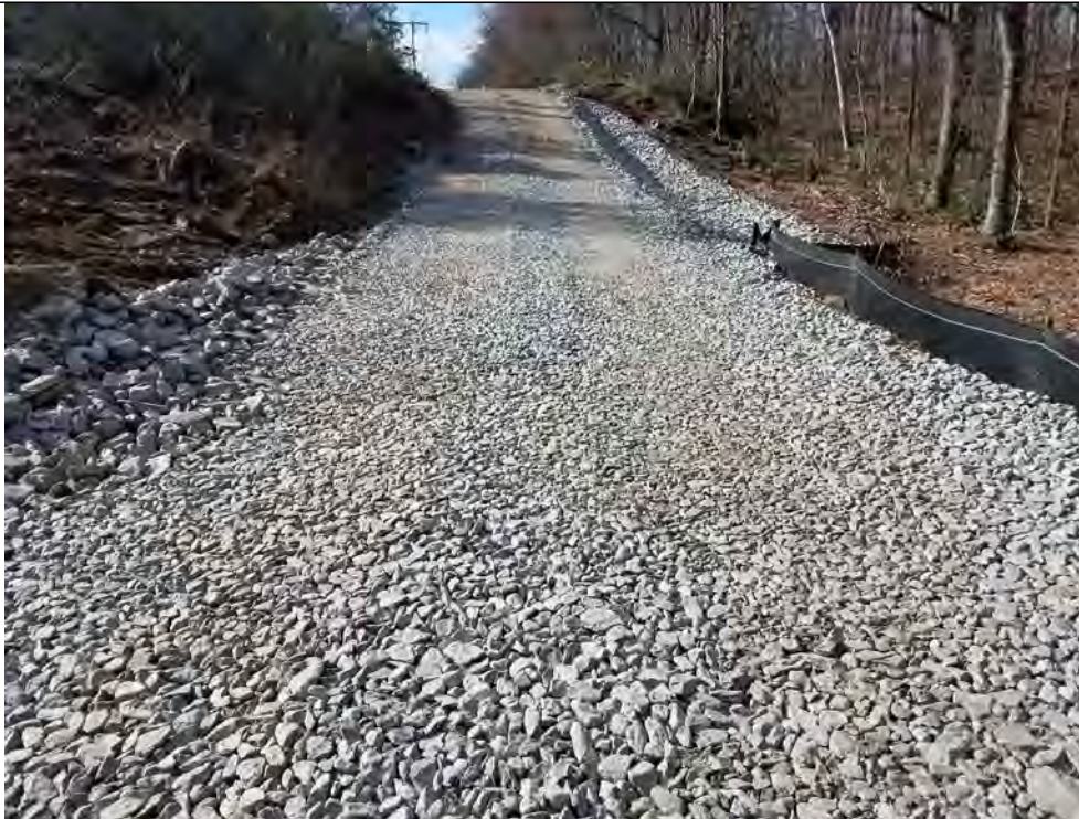
Photo 8: 4/14/2017, Watertown: Map 11, access road, water bar, stone swale and E&S improvements in the area of Str31.
