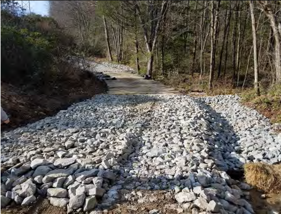
Photo 2: 4/14/2017, Watertown: Map 12, water crossing at W-C15 & S-C4, Stone access tracking pads and E&S Improvements.
