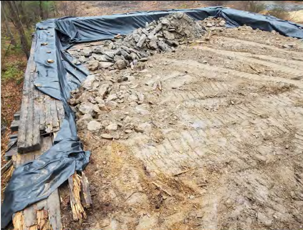
Photo 14: 4/21/2017, Thomaston: Map 18, construction of Str51 abutting W-D3 and S-D3.
