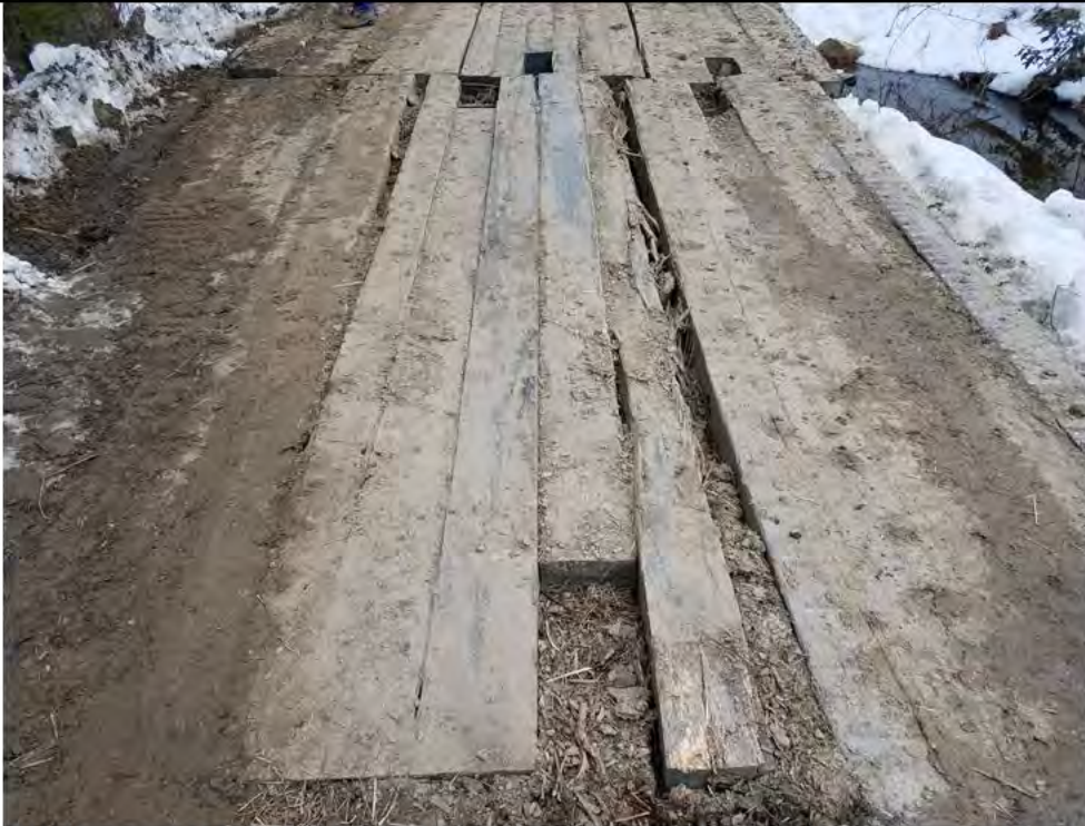
Photo 9: 3/24/2017, Watertown: Maps 09A-13, timber mat crossing, mat separation occurring at S-C4.
