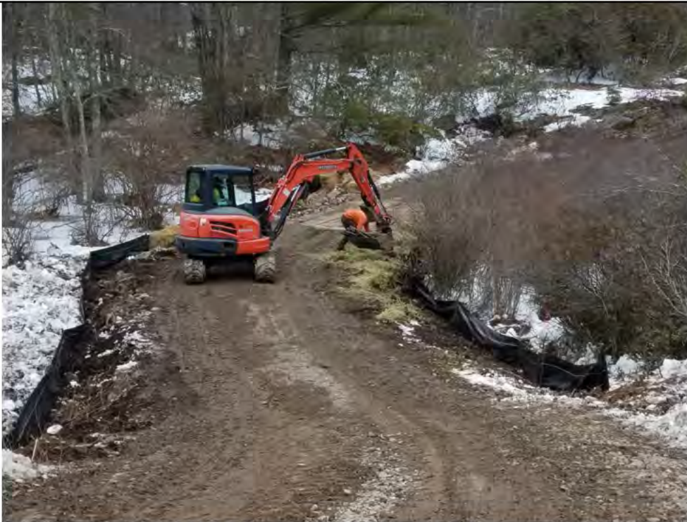
Photo 10: 3/24/2017, Watertown: Maps 09A-13, installing E&S at VP-C15-1.
