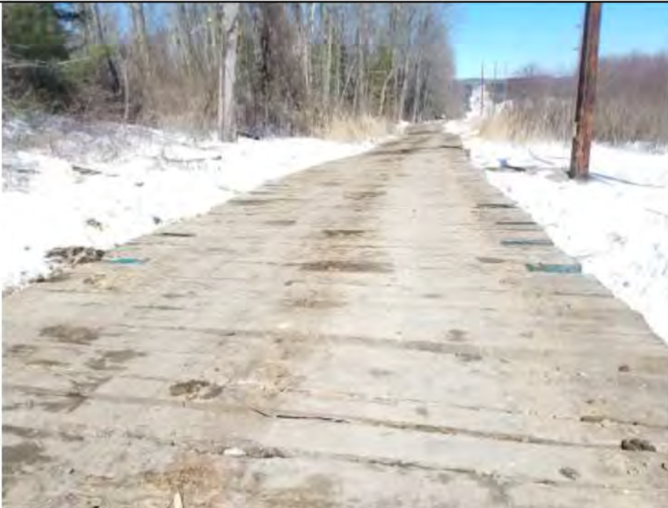
Photo 6: 3/17/2017, Litchfield: Maps 29 & 30, timber mat road through W-F7 to Str84.
