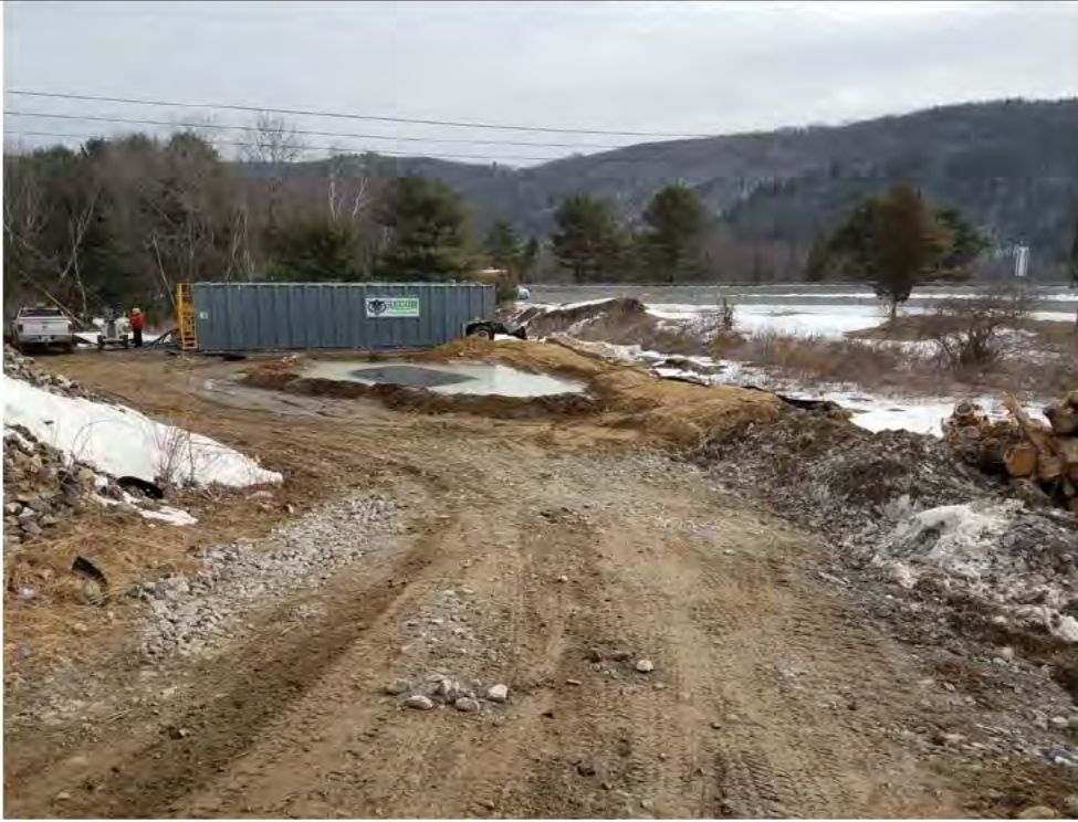
Photo 7: 3/24/2017, Watertown: Map 01, Str3080 and Str2, current dewatering set up (changes pending).
