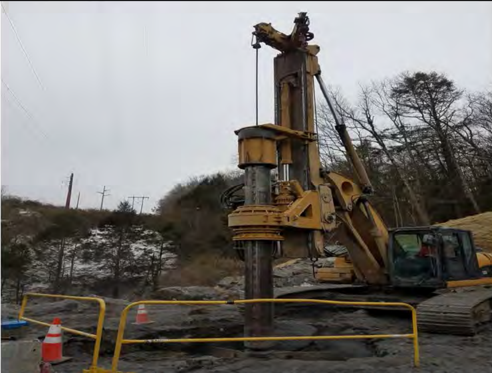
Photo 12: 3/24/2017, Litchfield: Maps 31 & 32, coring base for Vertical Deadend Structure, Str3171.
