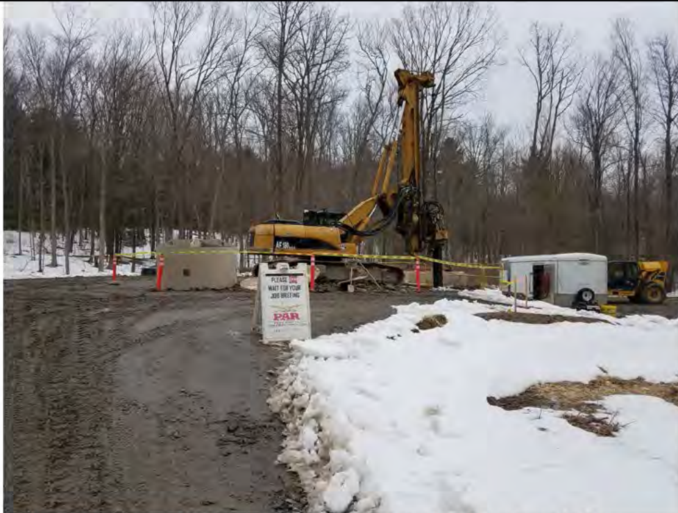
Photo 14: 3/24/2017, Harwinton: Map 35, coring base for Vertical Deadend Structure, Str96.
