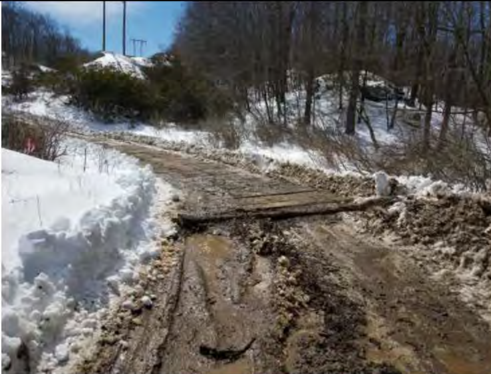
Photo 5: 3/17/2017, Watertown: Maps 09-13, timber mat at S-C4 crossing.
