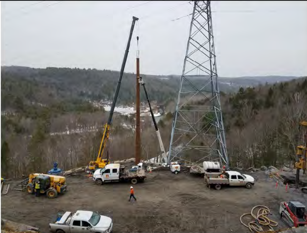
Photo 11: 3/24/2017, Litchfield: Maps 31 & 32, erecting Str86.
