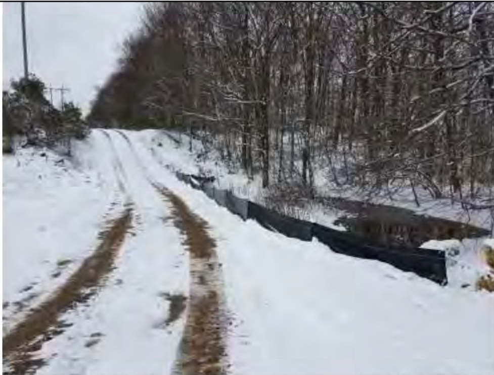
Photo 4: 3/10/2017, Thomaston: Map11, VP-C10-1, silt fence separating access road from vernal pool.
