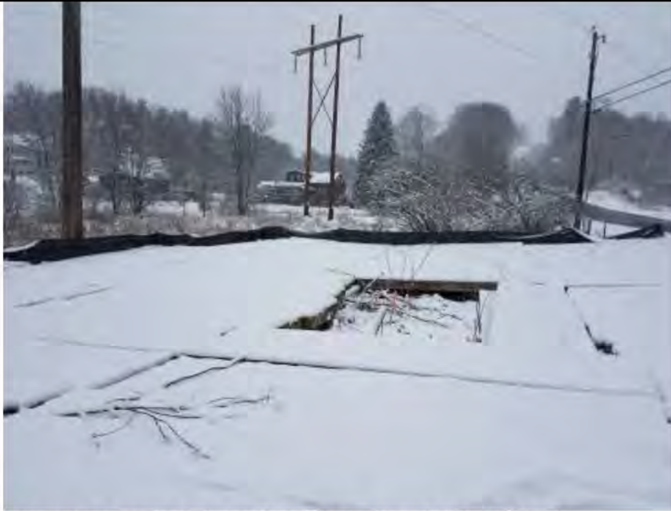
Photo 1: 3/10/2017, Harwinton: Map35, Str95, Silt fence placed around timber mat pad.
