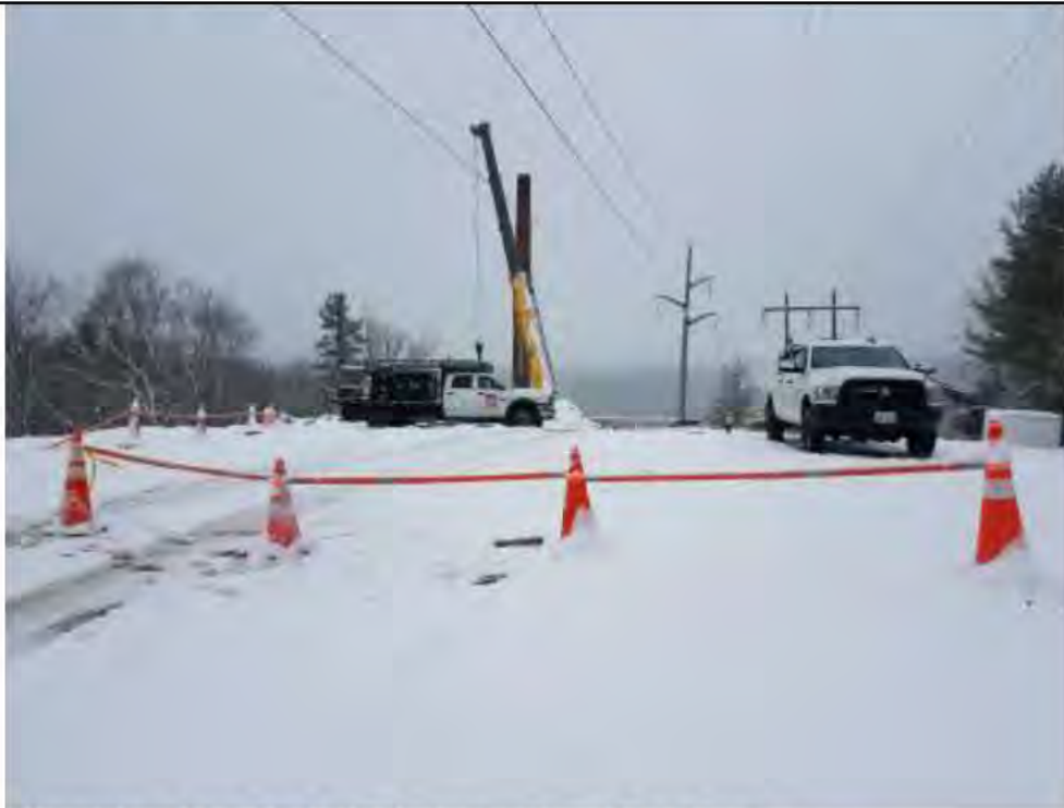
Photo 2: 3/10/2017, Harwinton: Map 32-34, Str88, construction of steel structure.
