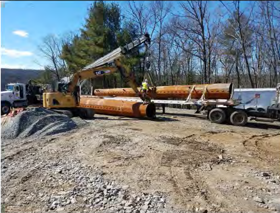
Photo 6: 3/3/2017, Harwinton: Map 32-33, Str88 delivery of typical structures pieces (Vertical Deadend).
