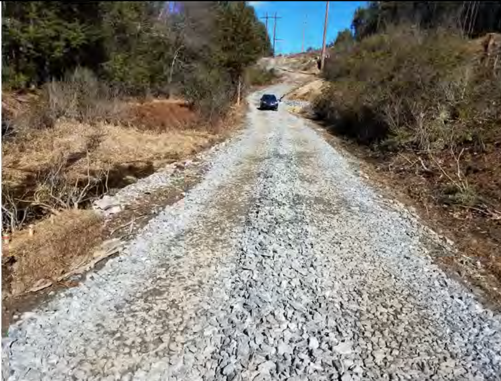
Photo 5: 3/3/2017, Harwinton: Map 32-33, Str88 access road improvements (grading and gravel placement).
