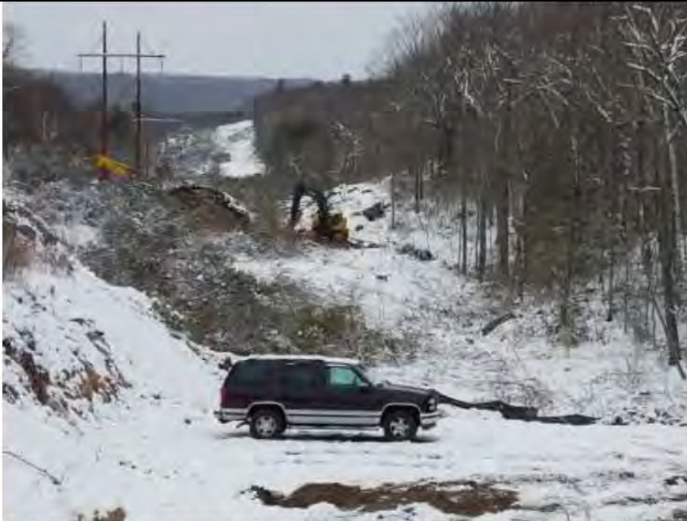
Photo 3: 3/10/2017, Thomaston: Map 25, Str70, mechanical clearing and pad construction.
