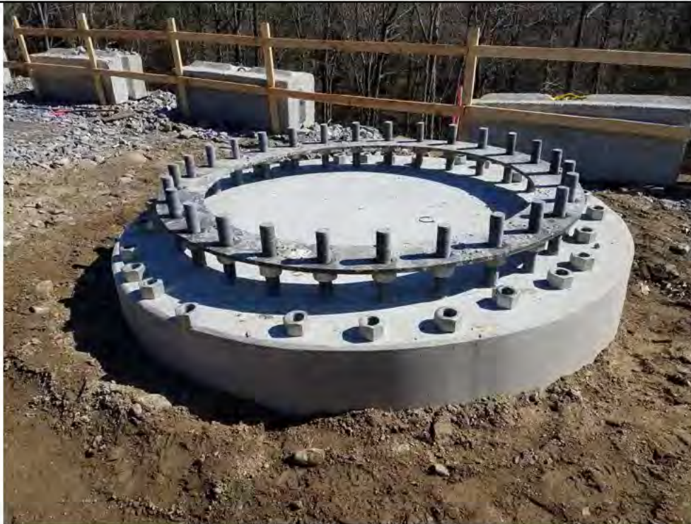
Photo 8: 3/3/2017, Harwinton: Map 32-33, Str88 finished drilled shaft foundation.
