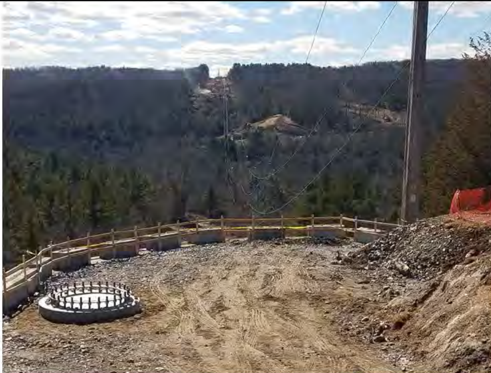
Photo 7: 3/3/2017, Harwinton: Map 32-33, finished Str88 pad and drilled shaft foundation.
